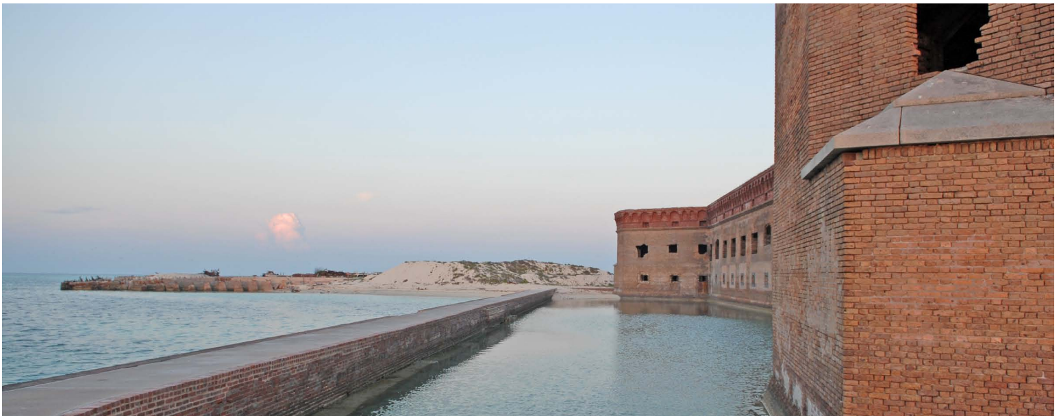
This moat at Dry Tortugas National Park is the last layer of protection between Fort Jefferson, a 19th-century coastal fortification, and sea level rise.
