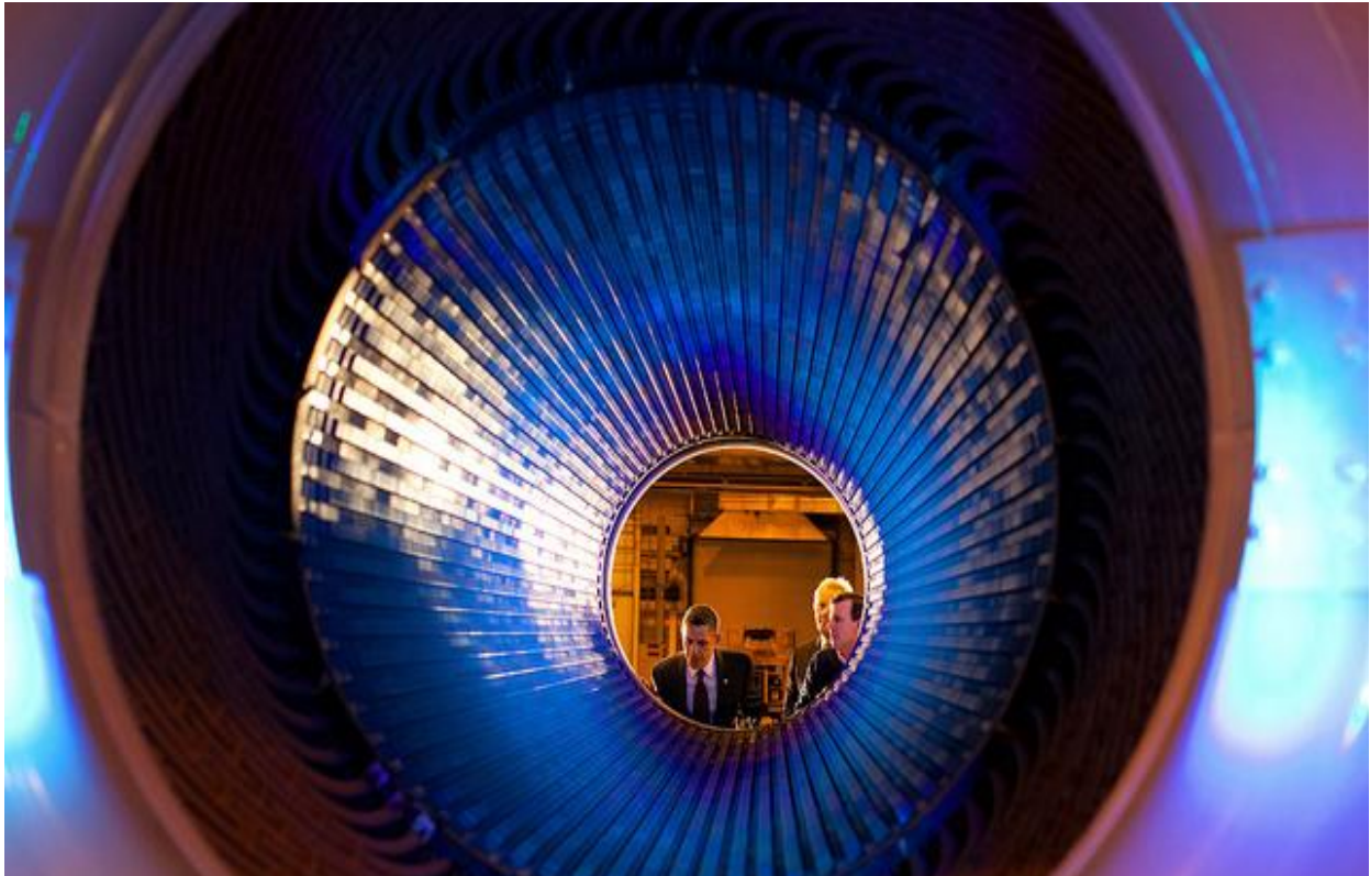
PRESIDENT BARACK OBAMA LOOKS INSIDE A HYDROGEN COOLED GENERATOR WHILE TOURING THE GENERAL ELECTRIC PLANT IN SCHENECTADY, N.Y., WITH GE CEO JEFF IMMELT AND PLANT MANAGER KEVIN SHARKEY, RIGHT, JAN. 21, 2011.
