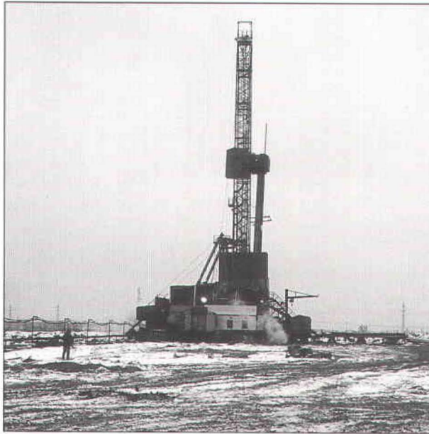
Drilling for oil in West Siberia.
