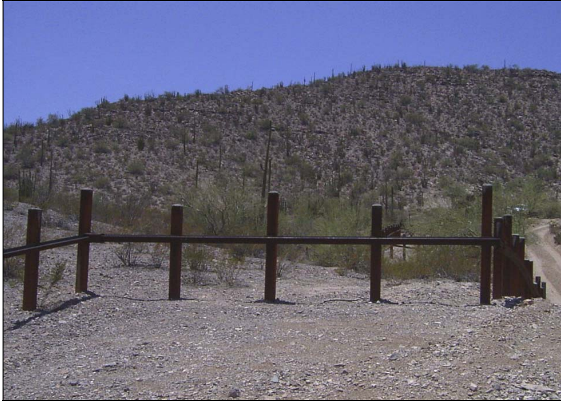
Figure 2-4. Photograph of Post-on Rail Fence
