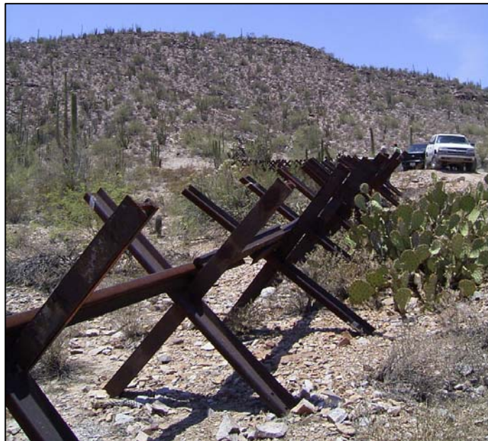
Photograph 1-2. Normandy Style Vehicle Fence
