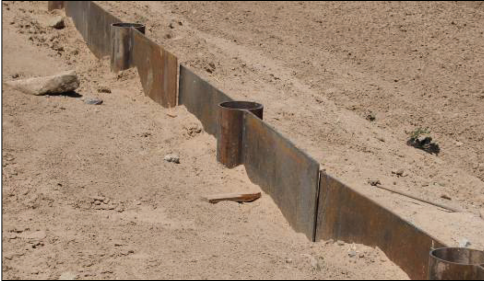
Figure A-1. Typical Primary pedestrian fence Foundation
