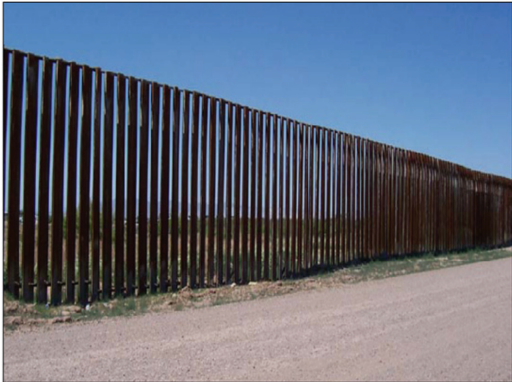
Figure A-7. Bollard Fence
