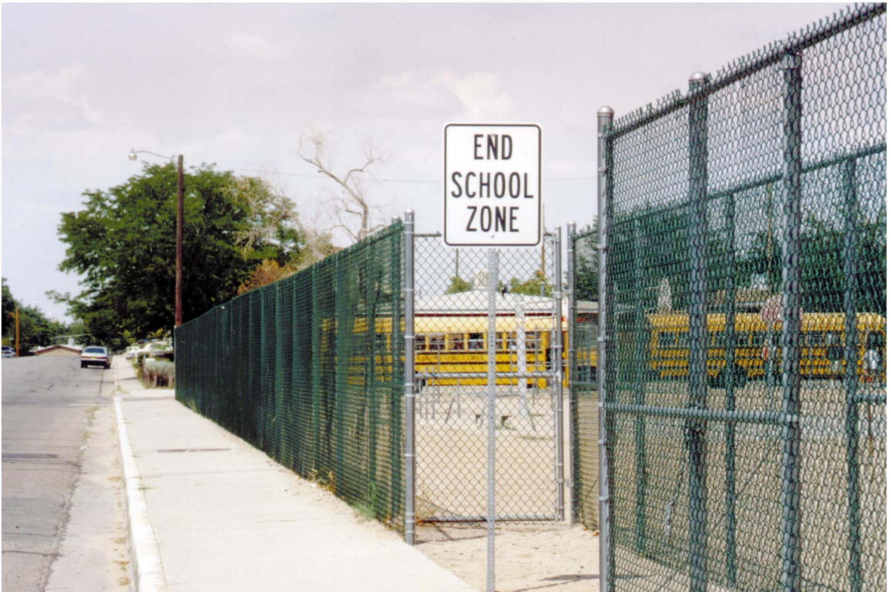
Exhibit 4.1. This 8-foot, small-mesh fence is around an elementary school. The school's problem with outside gang confrontations on the playground was completely eliminated.
