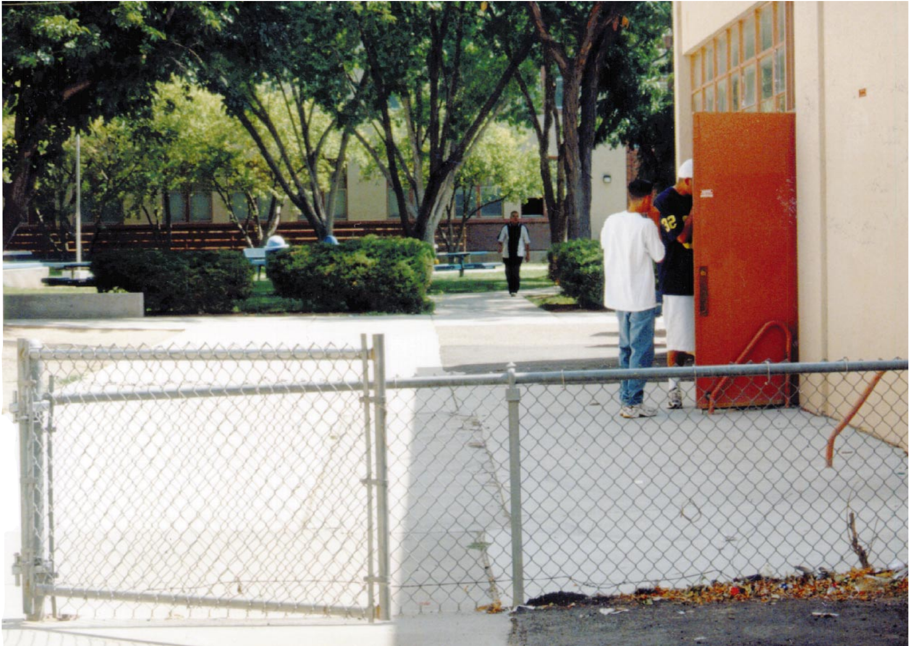
Exhibit 1.2. A 3-foot fence added very little security to this school that was constantly being vandalized.
