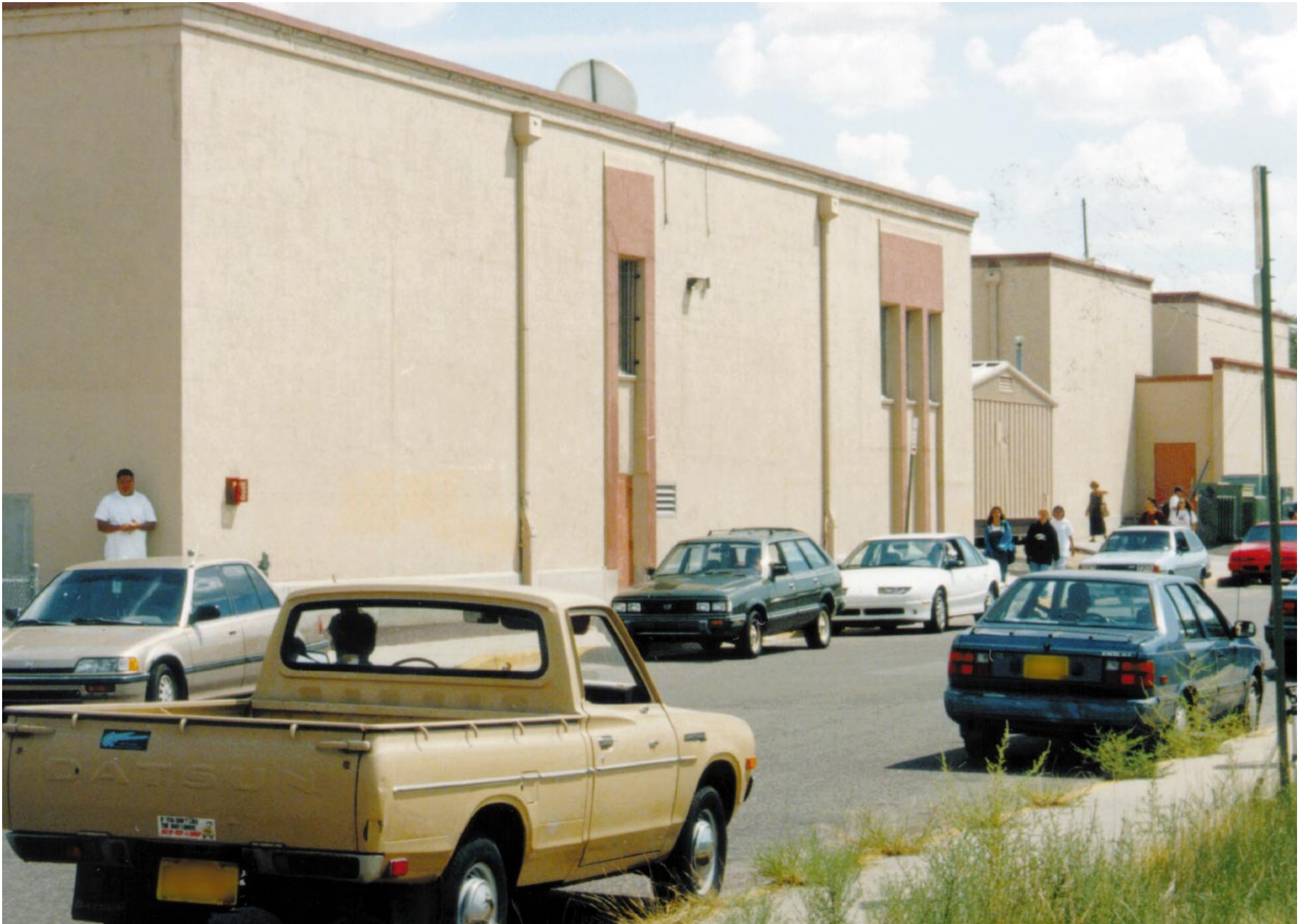
Exhibit 1.6. A school building's lack of setback from roads or parking areas can create vulnerability to an out-of-control vehicle.
