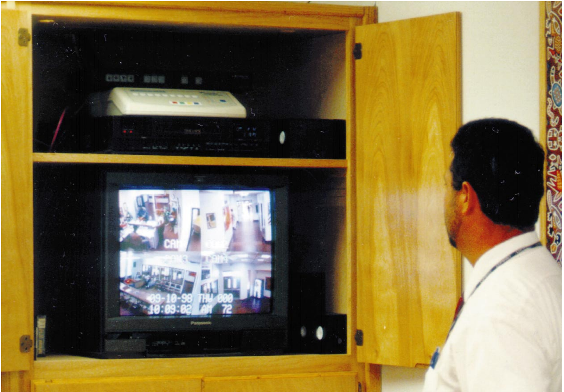
Exhibit 2.16. These monitors in the principal's office display the camera signals from the main entrance to Belen High School in New Mexico, and allow Ron Marquez to keep tabs on student entry and exit, even while he is in meetings.
