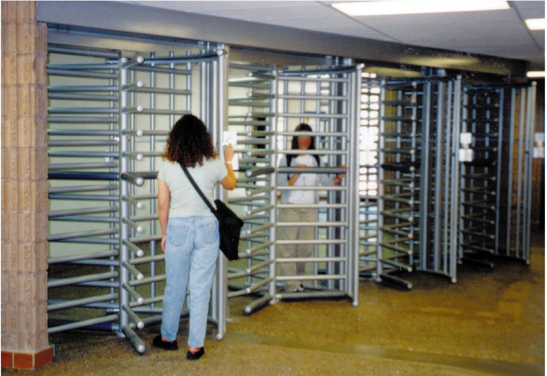
Exhibit 4.3. These turnstiles operate when a valid ID card is scanned through the card-swipe device; this type of arrangement can prohibit more than one person from entering with one valid card.
