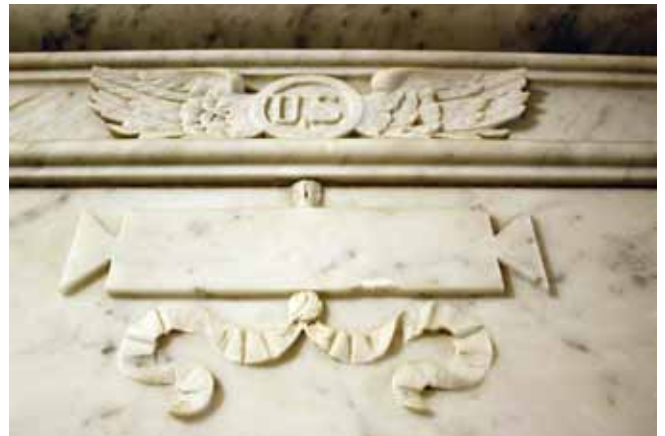
Customs Hall looking south, showing the restored skylight; carved detail on marble pilaster
