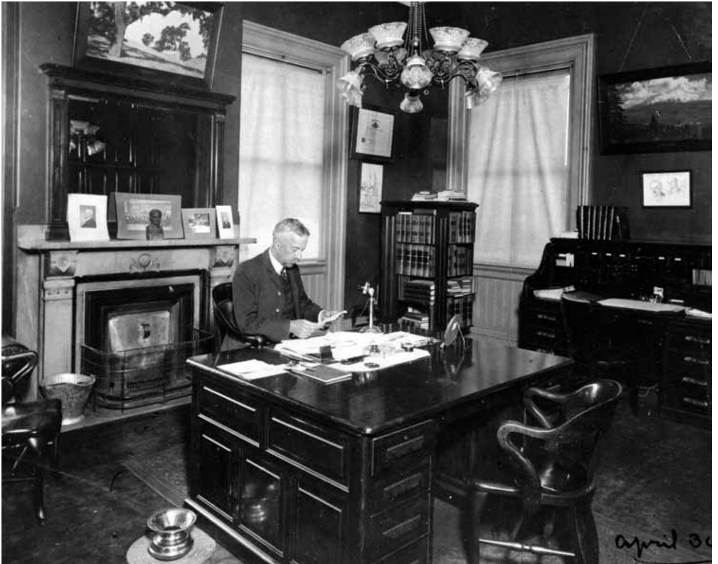
April 1909: Collector Frederick Stratton at work in his temporary quarters in the U.S. Appraisers' Building during construction of the new U.S. Customhouse
