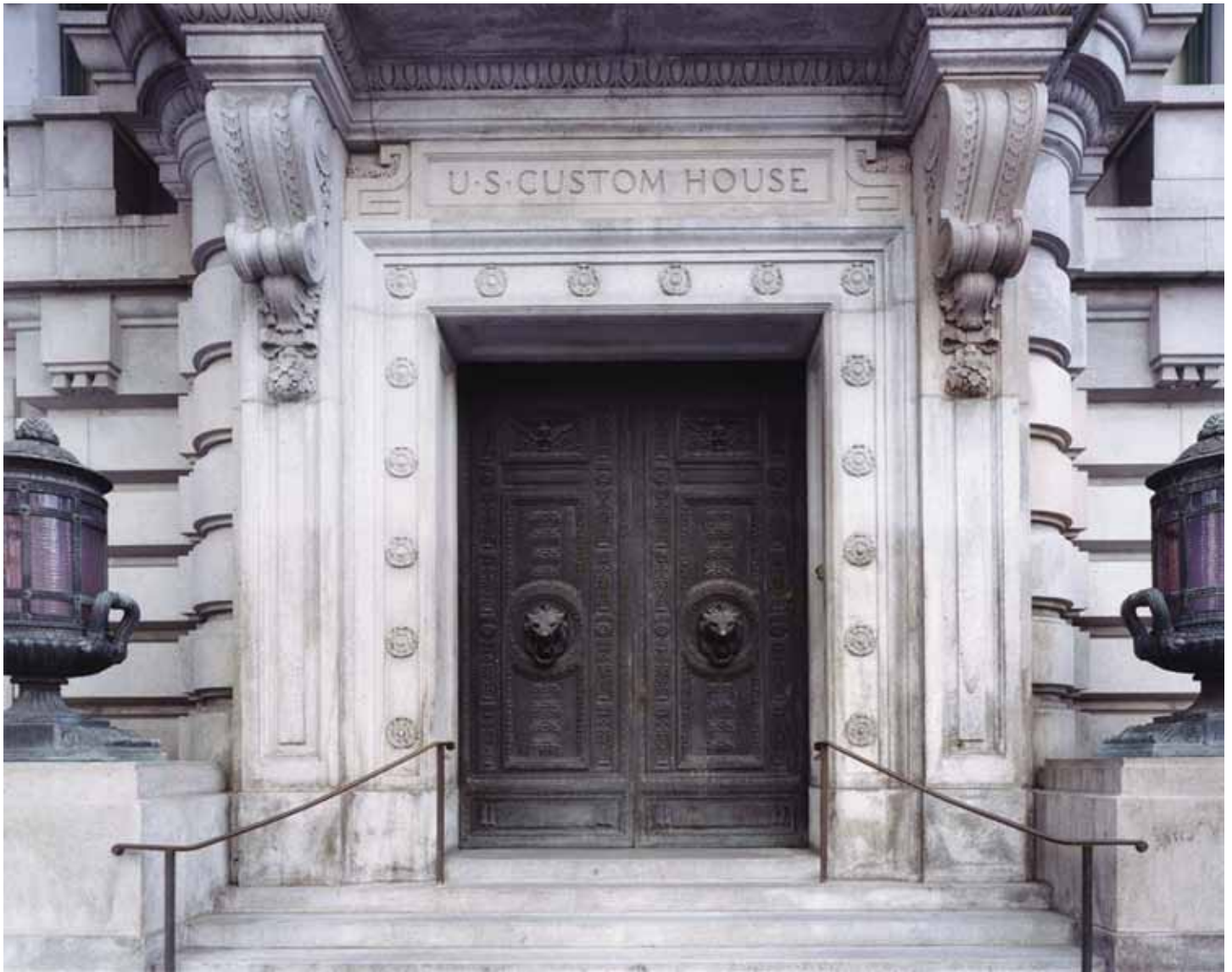
Above: Customhouse main entrance, Battery Street. Right: Customhouse view from Battery and Washington Streets.
