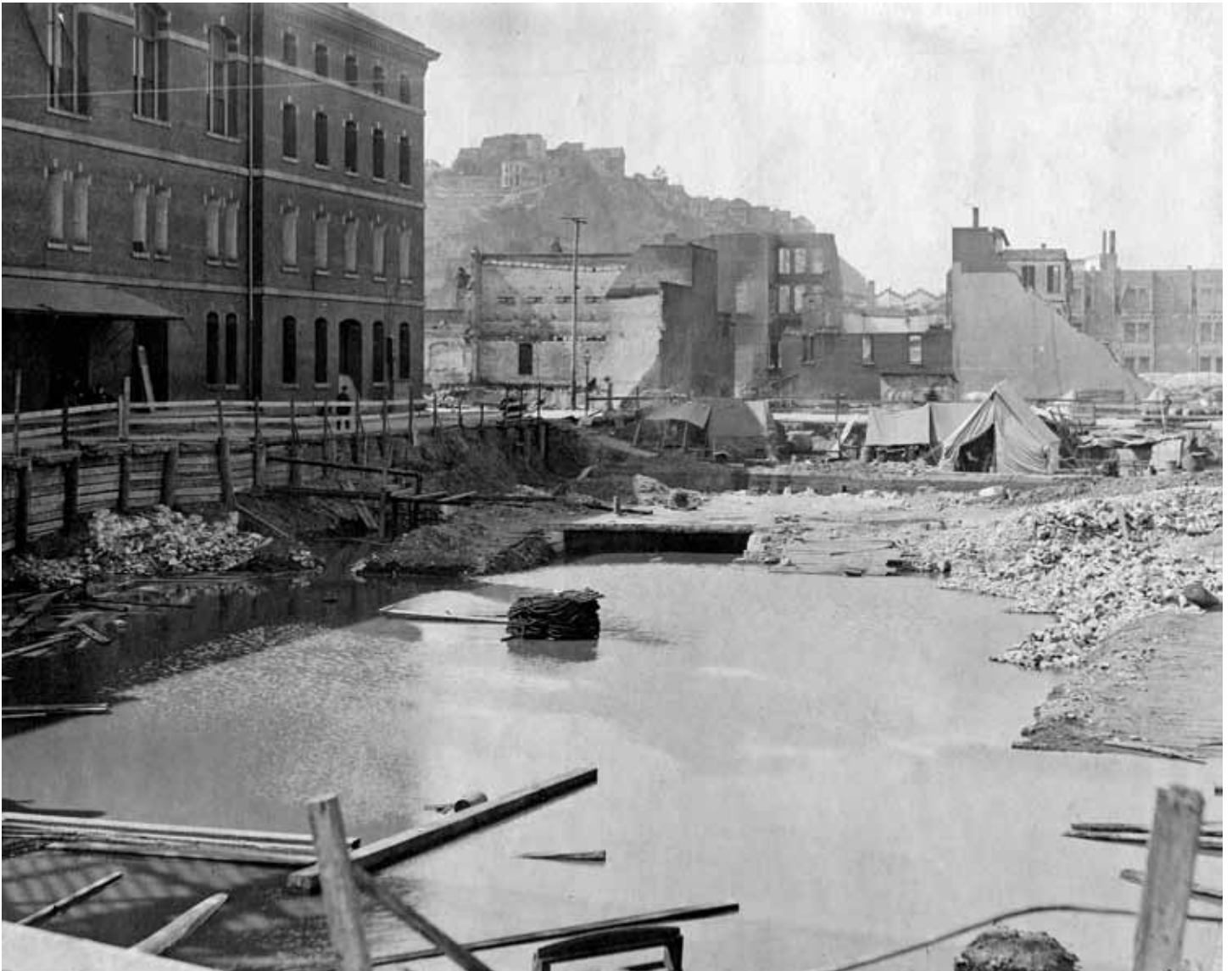
Seepage water from the excavated site of the demolished customhouse helped save the neighboring Appraisers' Building following the 1906 earthquake and fire
