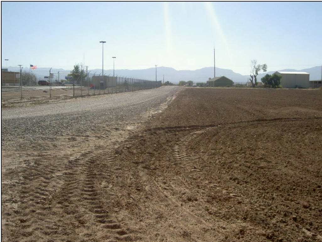
Photo 45. Fort Hancock Relay Tower Site, adjacent POE Station, facing southwest.
