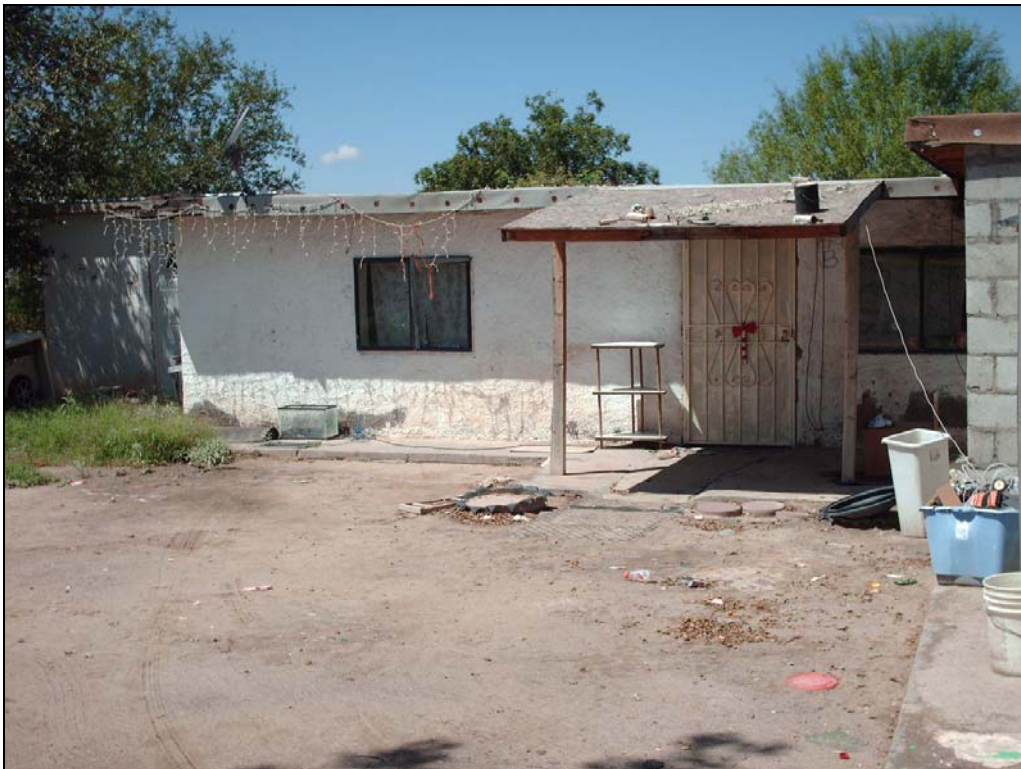
Photo 15. Tower Site EPT_FBN_071, facing west.
