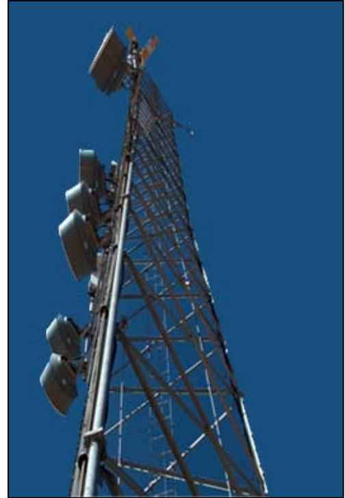
Photograph 2-1. Typical Surveillance and Communication Tower
