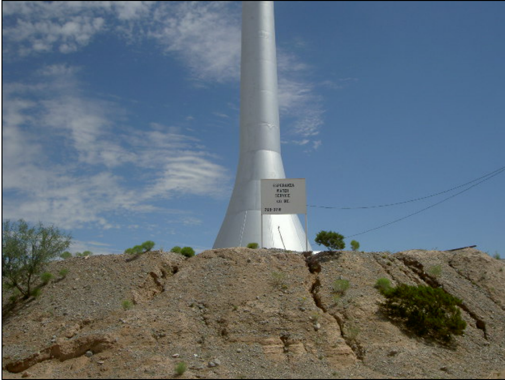
Photo 23. Tower Site EPT_FHT_069, facing north.
