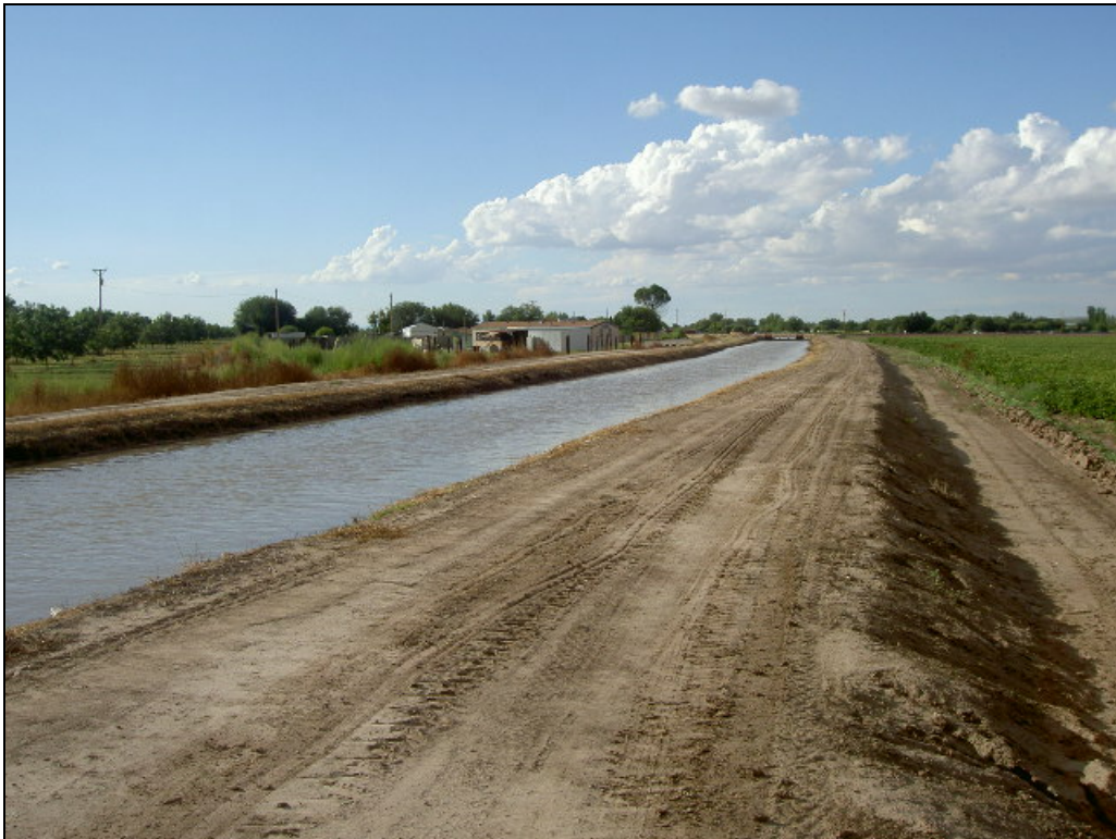
Photo 11. Tower Site EPT_FBN_056, facing west.
