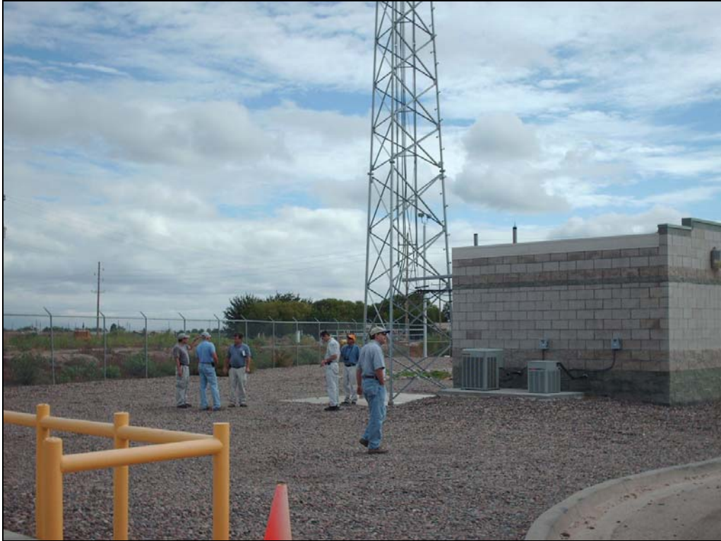
Photo 9. Tower Site EPT_FBN_055, facing southeast.
