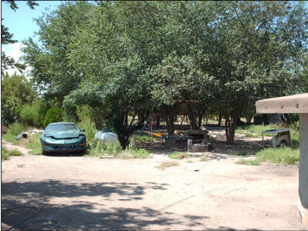
Photo 14. Tower Site EPT_FBN_071, facing south.
