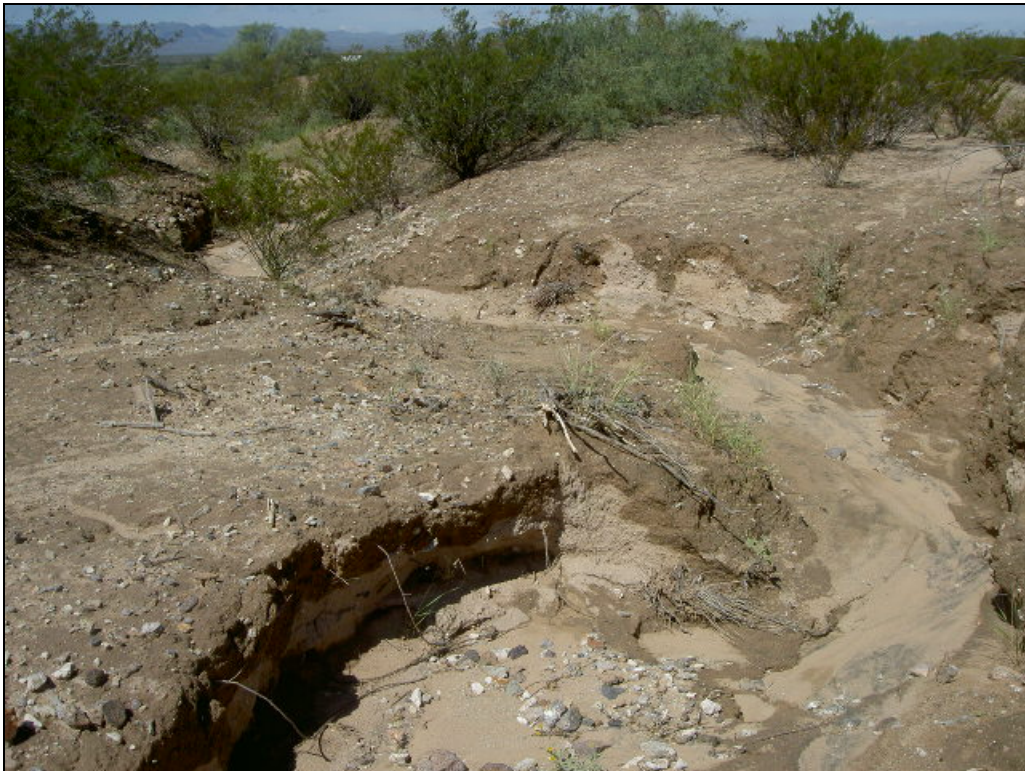
Photo 35. Tower Site EPT_FHT_068, wash crossing access, facing north.
