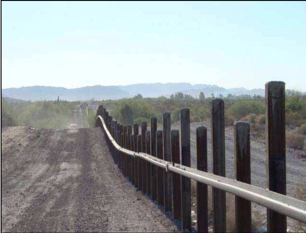
Figure B-1. Post-and-Rail Vehicle Fence (VF-1)
