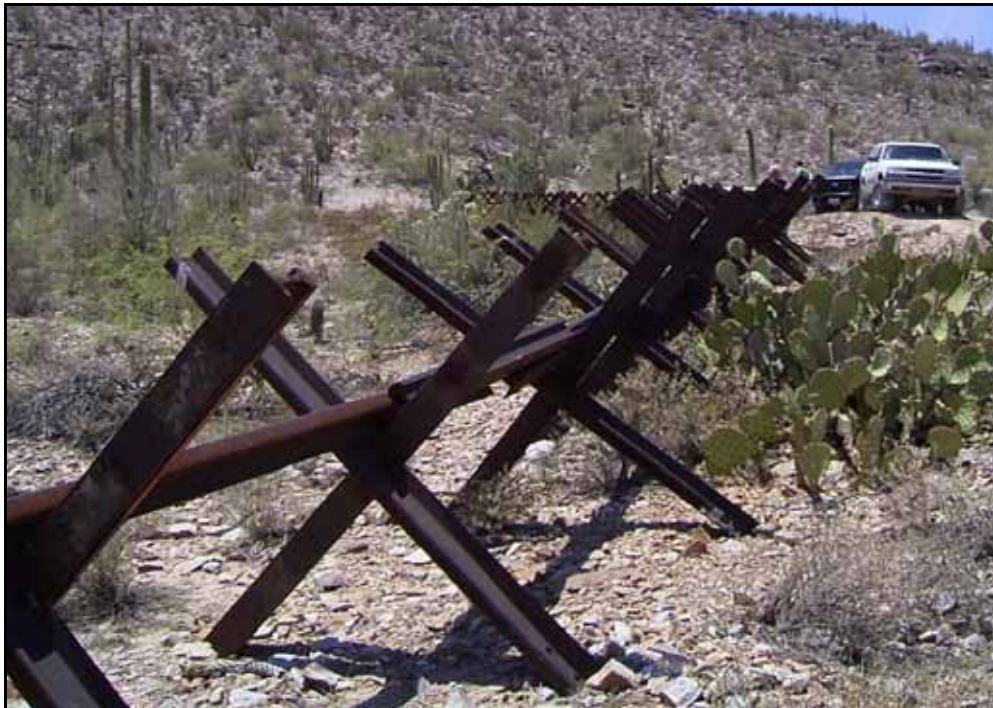
Figure 1-3. Normandy-Style Vehicle Fence (Fence Type VF-2)
