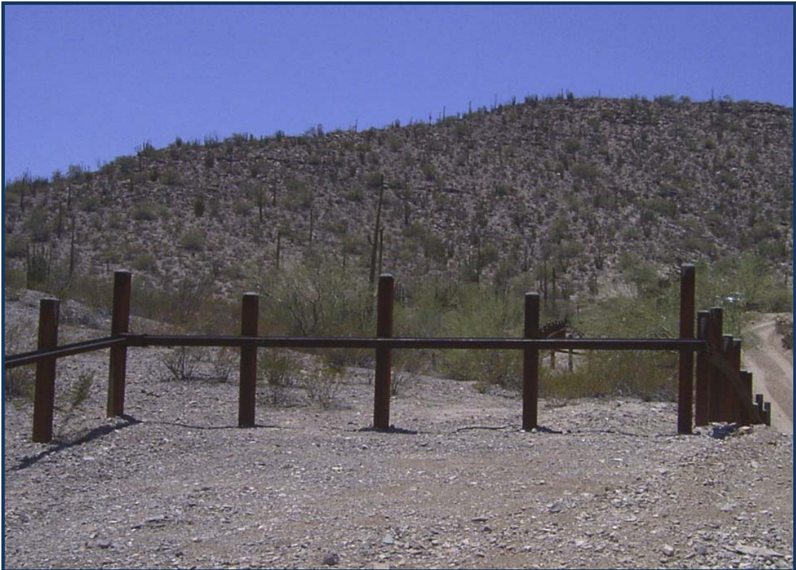
Figure 2-1. Photograph of Post-on-Rail Fence
