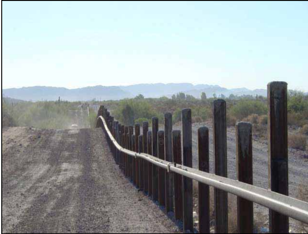
Figure 1-2. Post-on-Rail-Style Vehicle Fence (Fence Type VF-1)
