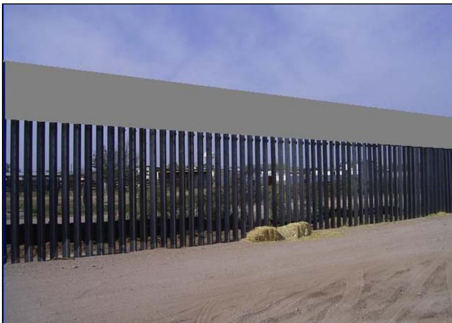
Figure 1-2. Personnel-Vehicle Fence Type-1 (PV-1)
