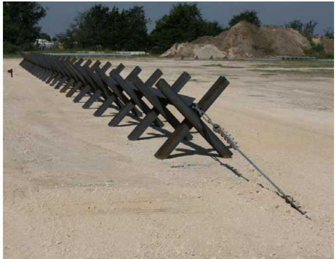
Photograph 2-2. Example of Normandy Style Vehicle Fence
