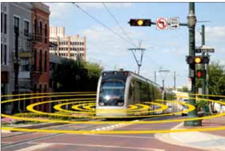
Houston, Texas, Metro, passenger train going through an intersection. ©iStockPhoto/Zellmer/US DOT
