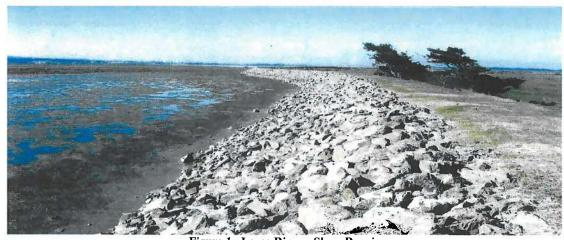
Figure 1. Levee Riprap Slope Repair Source: E&D consulting firm records for Project 2076
