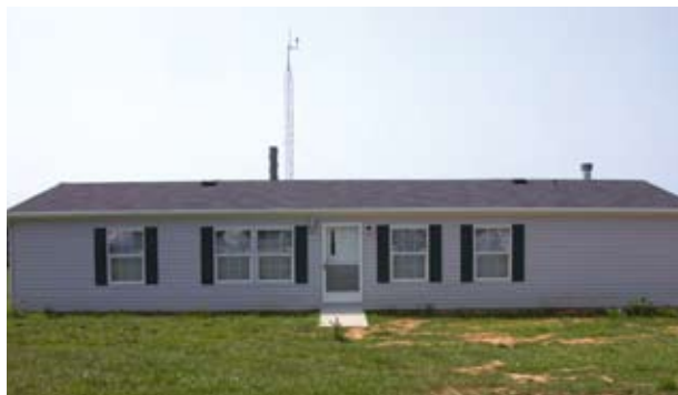
The Building Environment and Indoor Air Quality Test House is being used to study residential indoor air quality issues including exposure to ultrafine particles from common household activities, carbon monoxide poisoning associated with the operation of emergency generators, and whole house performance of air cleaning systems.
