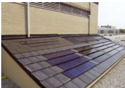
Six photovoltaic (PV) roofing products are currently being monitored to provide the data needed to develop, improve, and validate computer simulation programs that model the response of PV systems for a wide range of environmental conditions.
