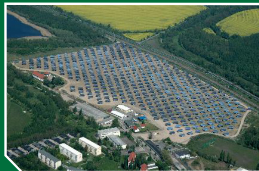
Today, 3.4 MW PV array (source: GEOSOL)
