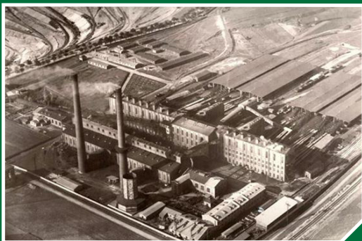
Former Borna briquette plant (source: GEOSOL)
