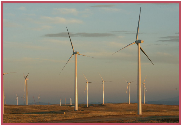
Turbines at the Glenrock wind farm in Wyoming. (source: PacifiCorp)
