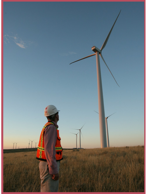
Glenrock wind farm in Wyoming. (source: PacifiCorp)
