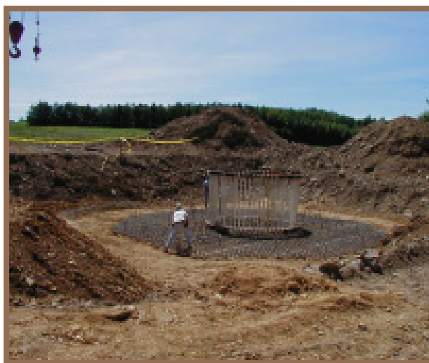
Step 2: Building each turbine's steel-reinforced concrete foundation.
