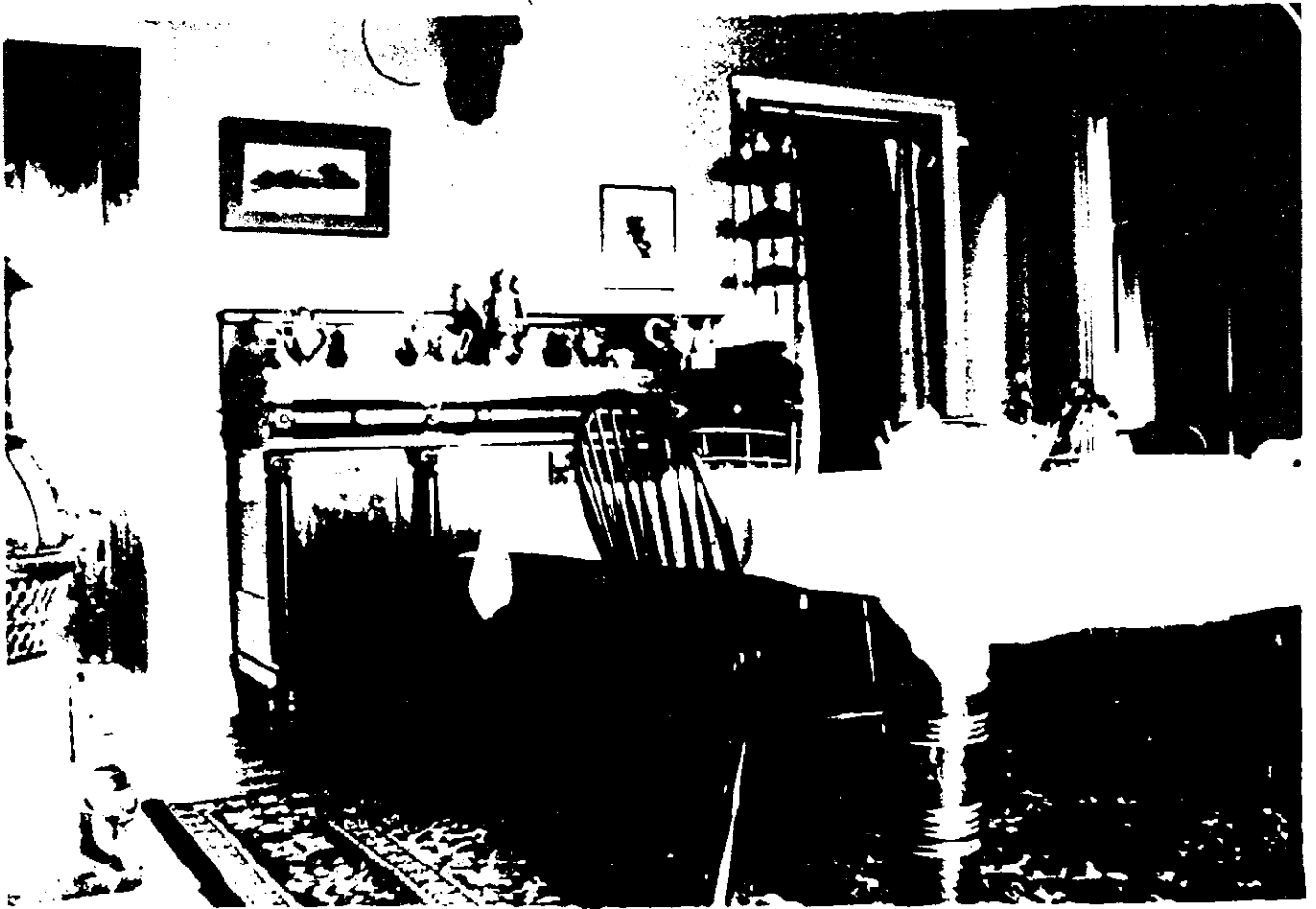
historic photograph, ca. 1900 dining room
