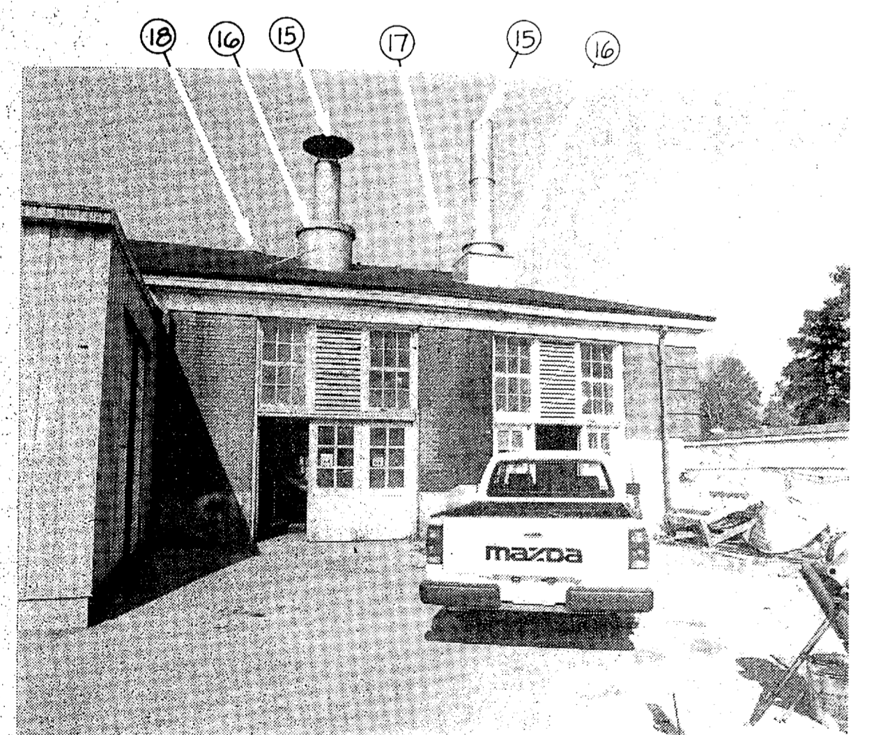
PHOTO-OUTSIDE BOILER ROOM (LOOKING NORTHWEST) NO SCALE
