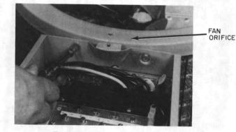
Fig. 3 - Removing Orifice Fan
