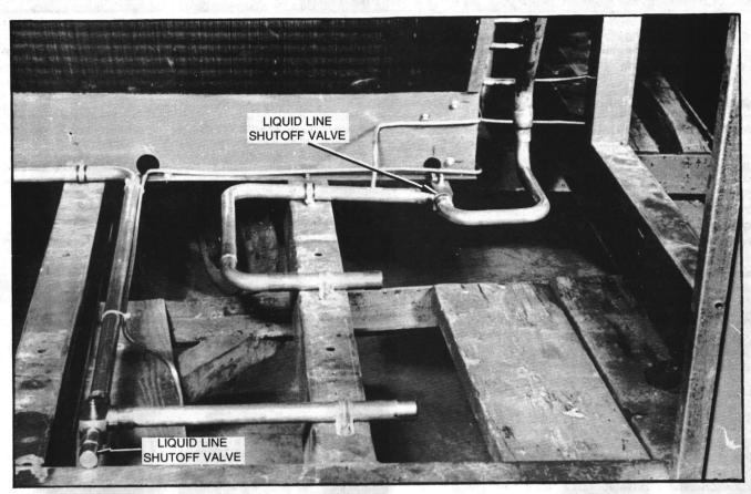
FIGURE 16 - Liquid Line(s) Piping (40, 50 and 60-Ton Units)
