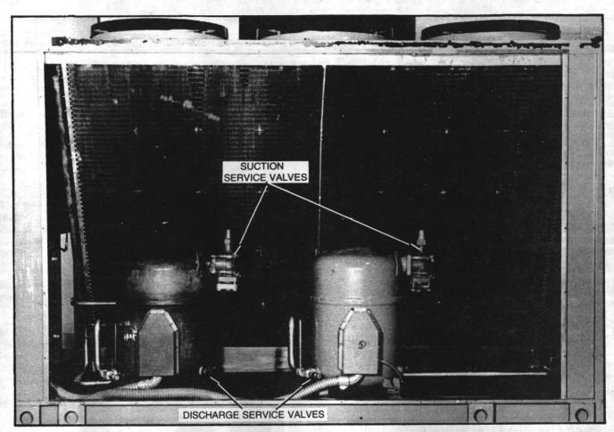
FIGURE 44 - Compressor Access Valves
