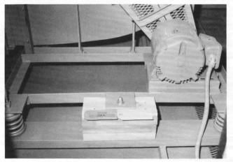
Backward Curved Fan With Belt Guard and Spring Isolators
