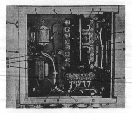
1 Wet well alarm switch Wet well alarm indicator light 2 Wet well alarm buzzer 3 Solution feeder circuit breaker 4 5 Wet well alarm circuit breaker Agitator drive motor circuit breaker 6 7 120 volt outlet circuit breaker 8 120 volt outlet
