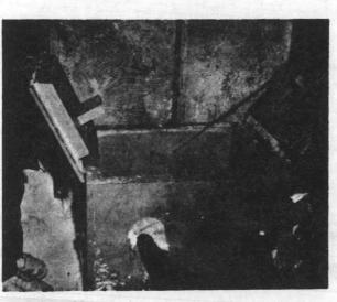
Fig 1-28. Insulated box for raw water pump.
