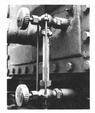
Fig 2-39. Evaporator distillate gage.
