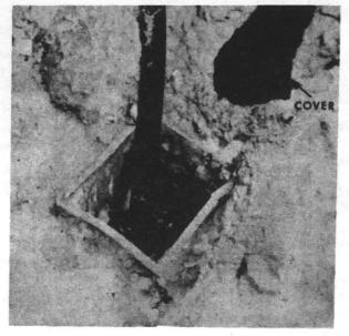
Fig 1-27. A method of protecting the intake point from freezing.
