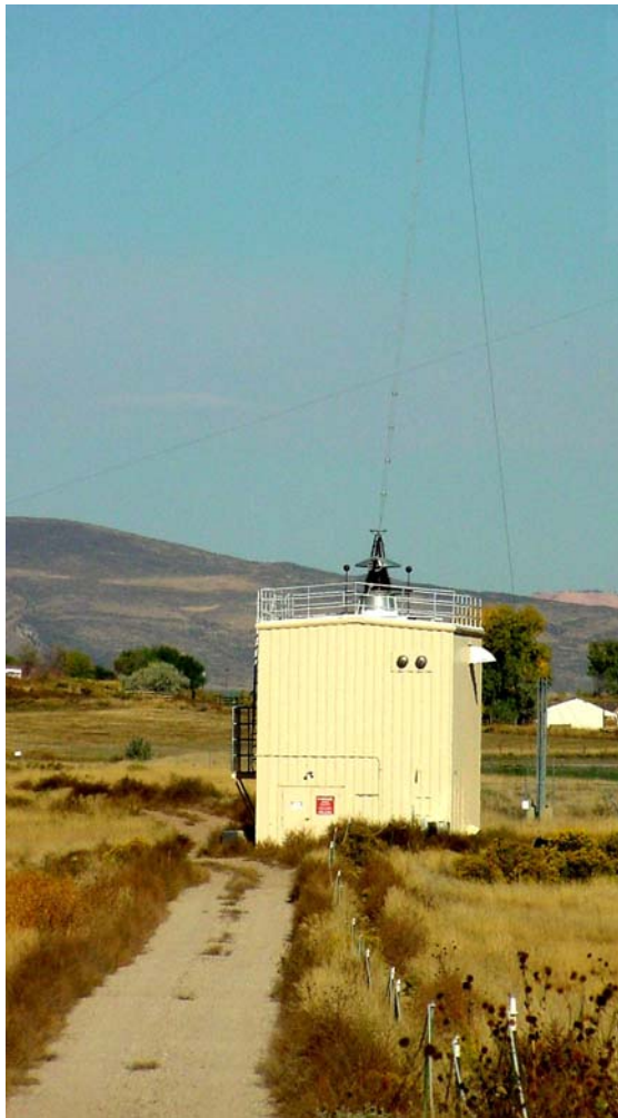
Figure 1.15. WWVB helix house.
