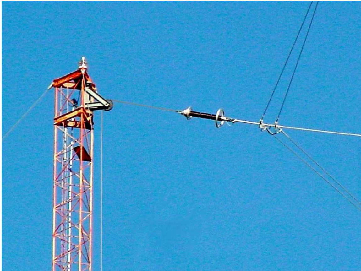
Figure 1.20. Antenna to tower connection detail.
