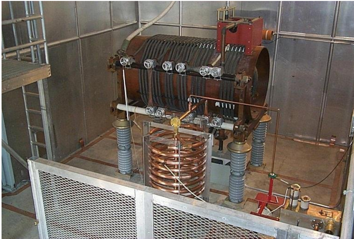
Figure 2.18. Interior view of helix house.
