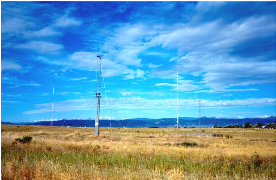
Figure 1.10. The 15 MHz antenna at WWV.
