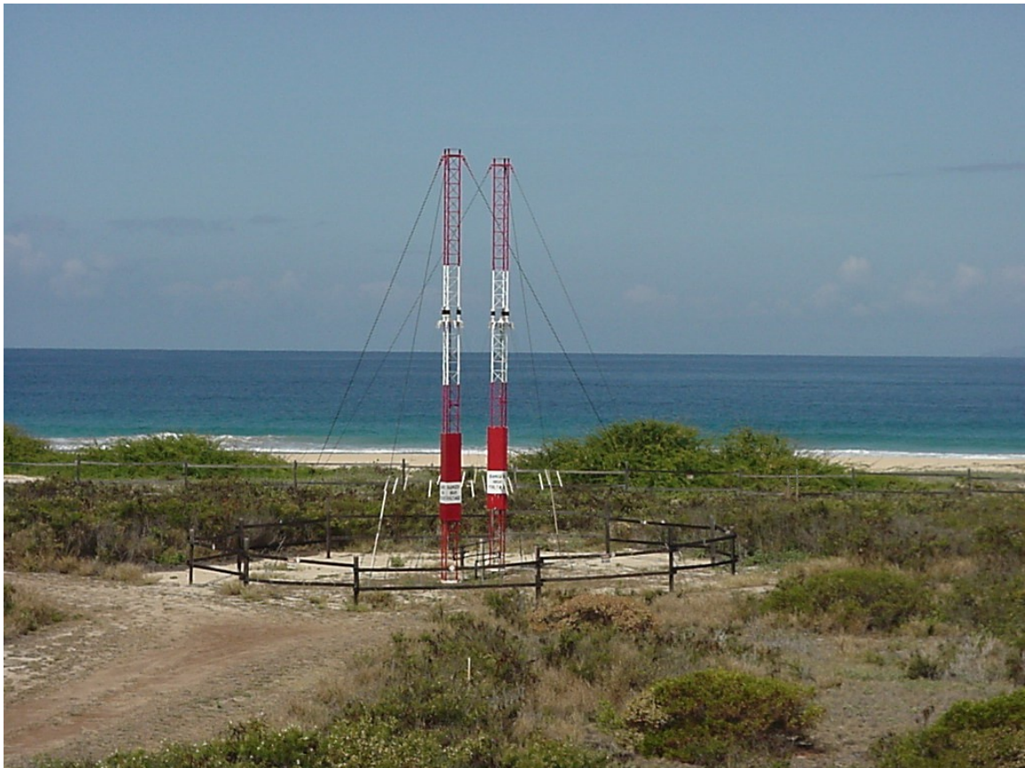
Figure 1.29. 15 MHz antenna at WWVH.
