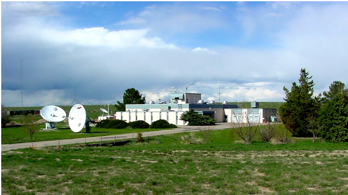
Figure 1.6. The WWV transmitter building.
