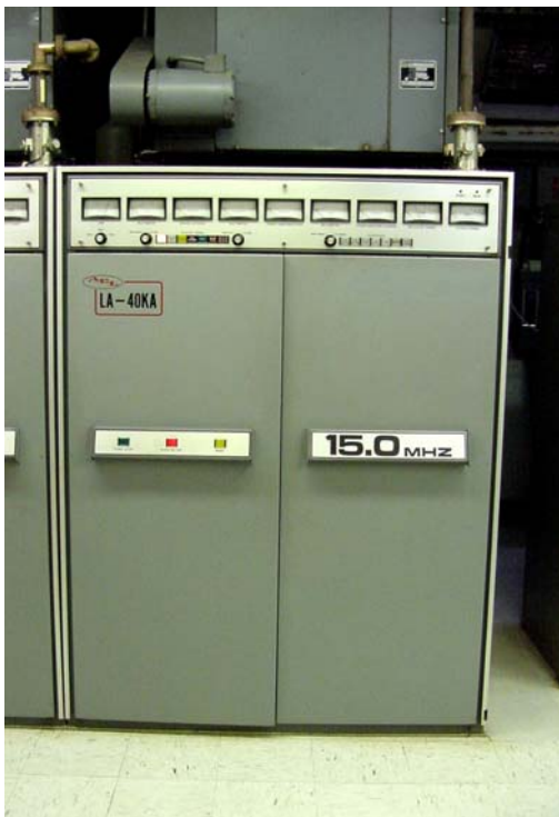
Figure 1.26. The 15 MHz standby transmitter at WWVH.
