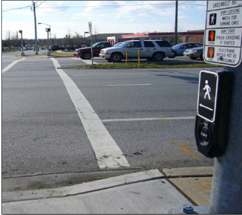
Figure 10: Location where tactile arrow is aligned with direction of travel on the crosswalk.
