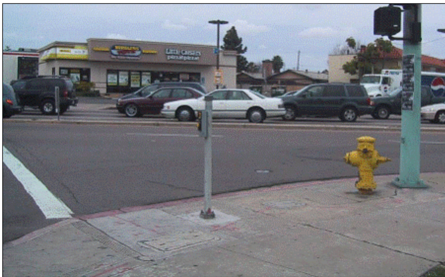
Figure 16: Stub pole was installed to locate APS near the crosswalk.
