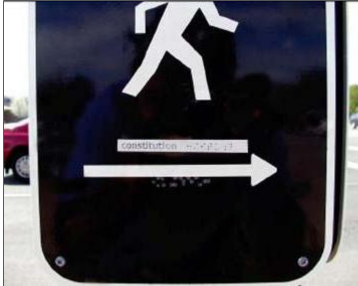
Figure 14: Braille sign installed backwards, with manufacturers' label showing. Label includes street name and print of how Braille should look. Braille beneath arrow is backwards version of the print version shown on label and is indented, rather than raised.
