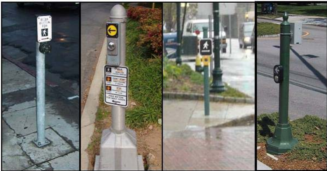
Figure 17: Examples of stub poles – different materials and installation.
