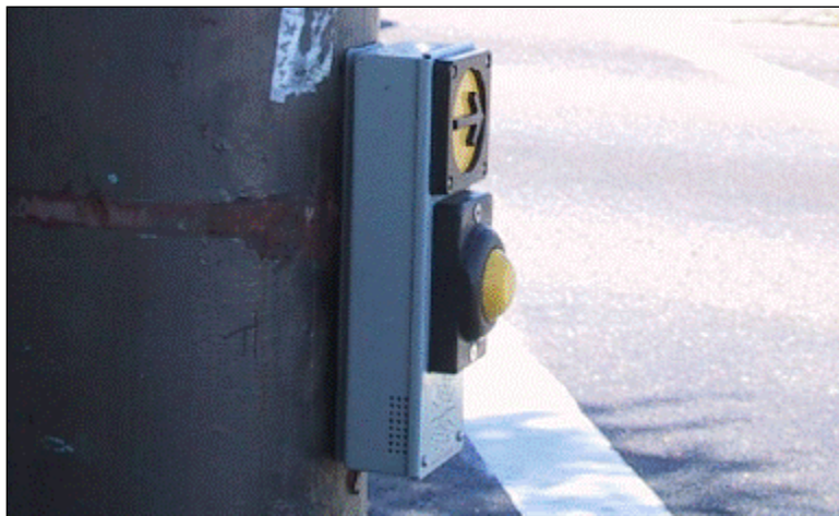
Figure 9: Tactile arrow not aligned with crosswalk direction.
