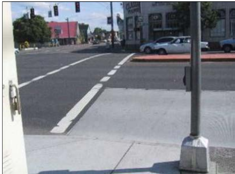
Figure 5: APS is located about 8 feet from the crosswalk and curb ramp landing.
