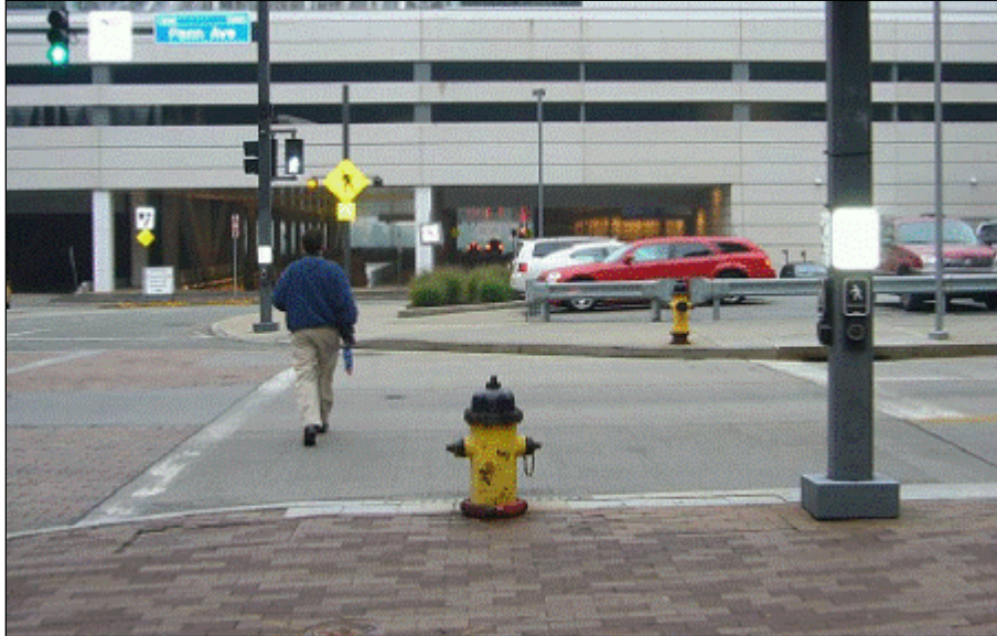
Figure 15: APS is located on mast arm pole more than 10 feet outside the crosswalk lines. In addition, a fire hydrant is between the crosswalk location (and the curb ramp) and the APS.
