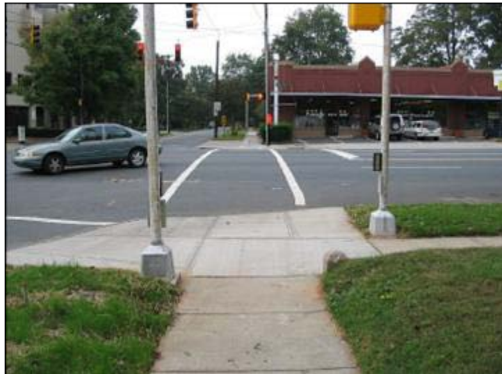
Figure 13: APS installed on poles in the landscape strip, and still within reach from a level paved sidewalk surface.
