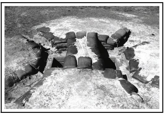
Figure 6-15. Two-man fighting position with built-up OHC (Stage 4).
