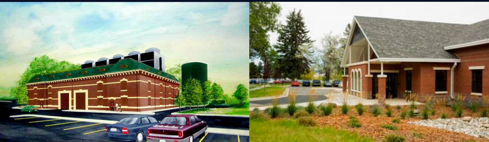
Bio-mass energy plant at Mountain Home (TN) VA Medical Center; Fort Harrison (MT) Regional Office – LEED certified building
