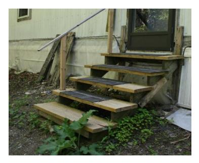
The picture above shows the rear steps, which needed a protective railing on the right side, and the landing at ground level, which was sloped, causing a tripping hazard.
