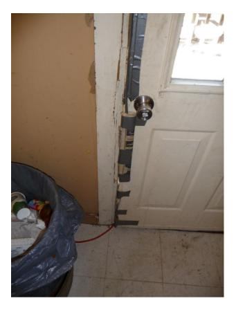
The picture above shows that the main entry door frame was separated and the door did not close correctly, as duct tape was used to hold it in place.
