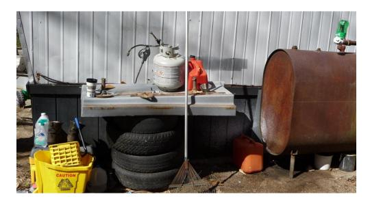
The picture above shows a 5-gallon portable propane tank located at the rear of the unit, which was connected to the kitchen stove. The propane tank was on top of a flat plastic container supported by four rubber vehicle tires near a gas can and an oil tank, which was a potential fire hazard.
