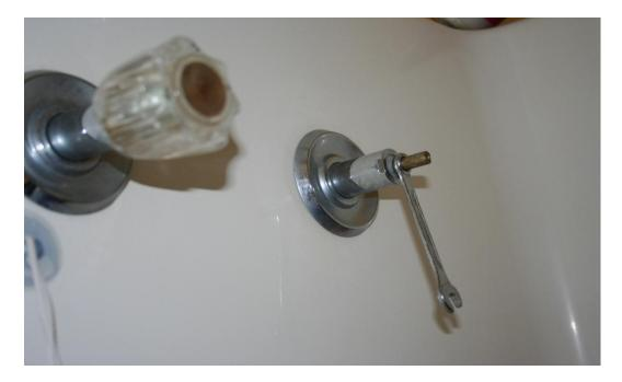
The picture above shows that the tub-shower was missing a control handle and a wrench was being used as a substitute.
