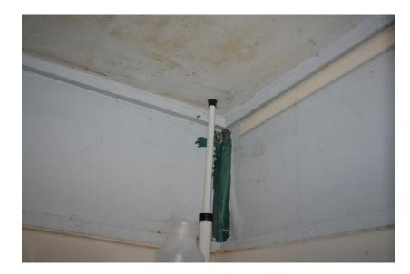
The picture above shows mold and mildew on the ceiling and a hole in the corner of the shower area that was taped and could lead to water damage.
