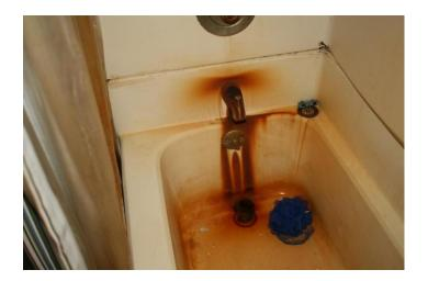
The picture above shows a rust-stained tub that was preexisting and should have been replaced or repaired. The tub is a health and safety issue.
