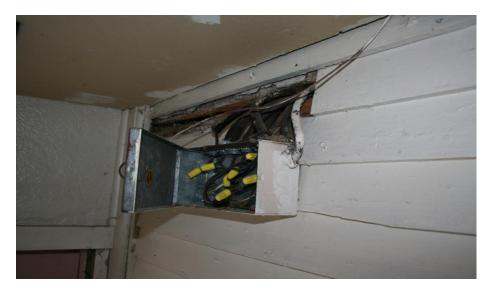
The picture above shows a preexisting electrical issue of wiring coming from a hole in the wall into a junction box that was not secured, exposing more wire in the foyer-entrance to a unit.
