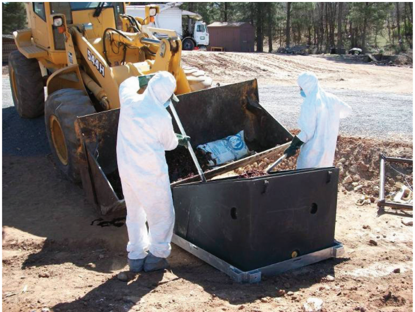
Figure 1. Employees in PPE shoveling material from a pit toilet into a backhoe clamshell shovel.
