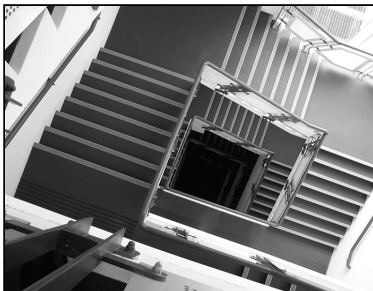
Figure 7-42. Enclosed stairwell (large gap)
