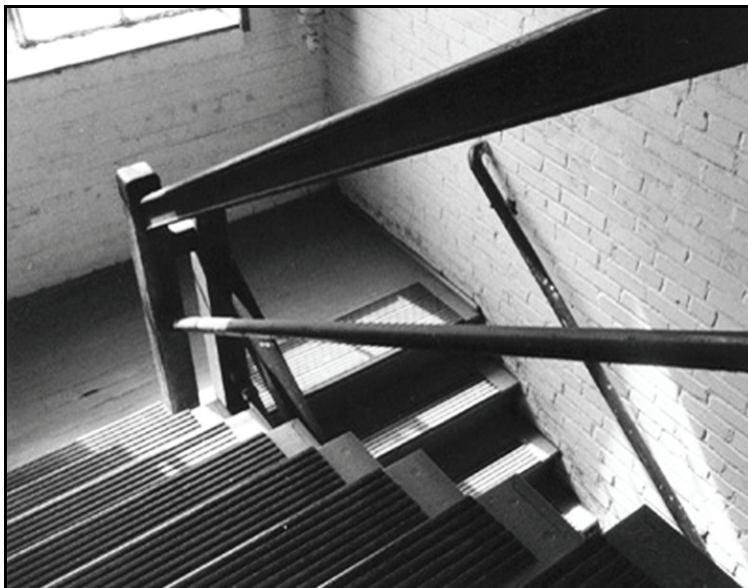
Figure 7-41. Enclosed stairwell (small gap)
