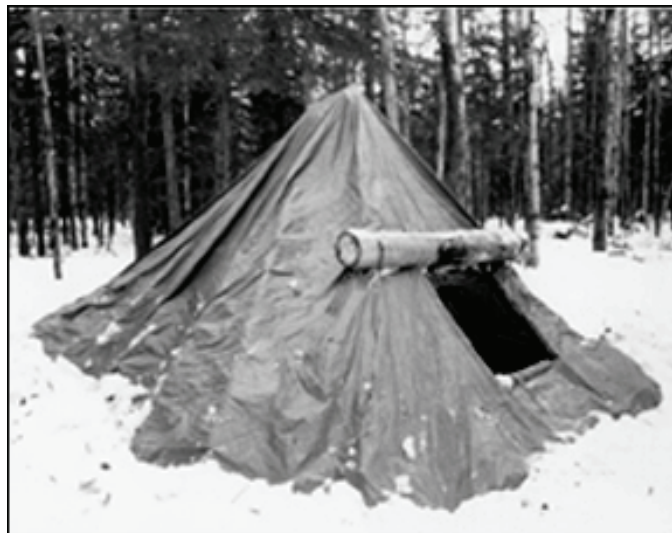
Figure 2-2. Covered frame of infrared counterdetection (thermal) shelter
