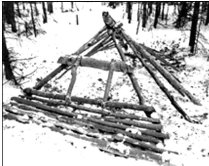
Figure 2-1. Frame of infrared counterdetection (thermal) shelter
