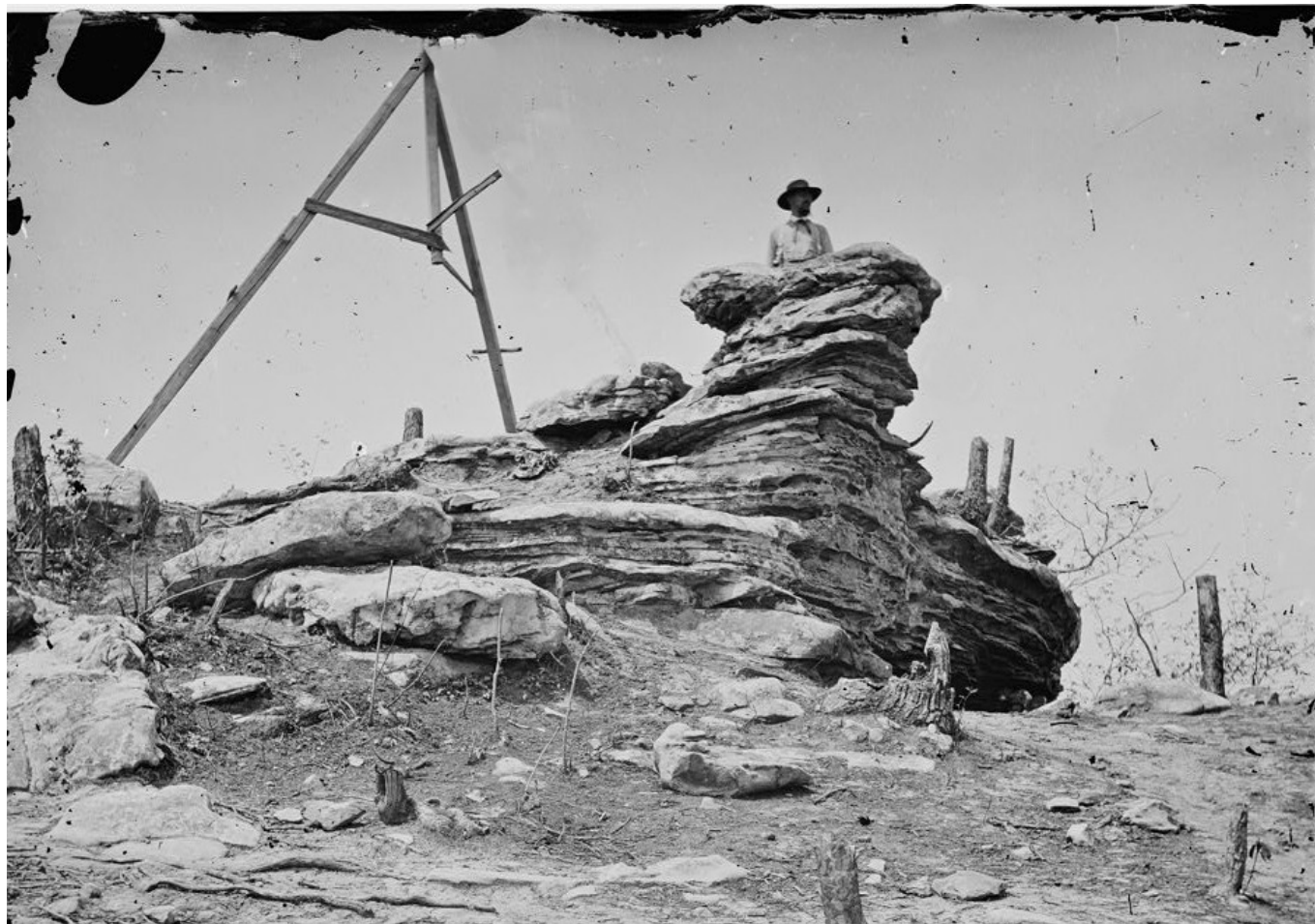
Tripod signal erected by Captains Dorr and Donn of U.S. Coast Survey at Pulpit Rock on Lookout Mountain after it was captured by Union troops.
