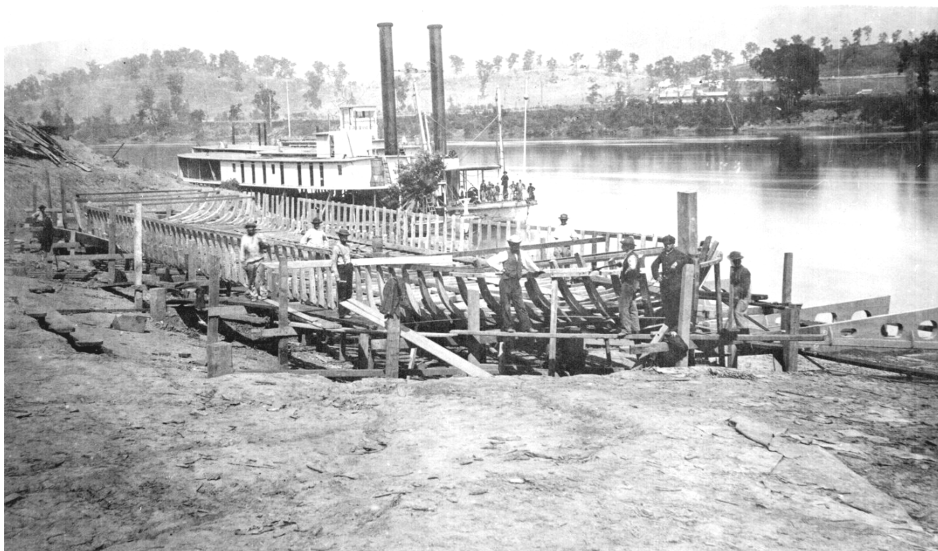
U.S. Army Engineers build the steamboat Chattanooga (background) on the banks of the Tennessee river during the siege. Another steamboat is under construction in the foreground.
