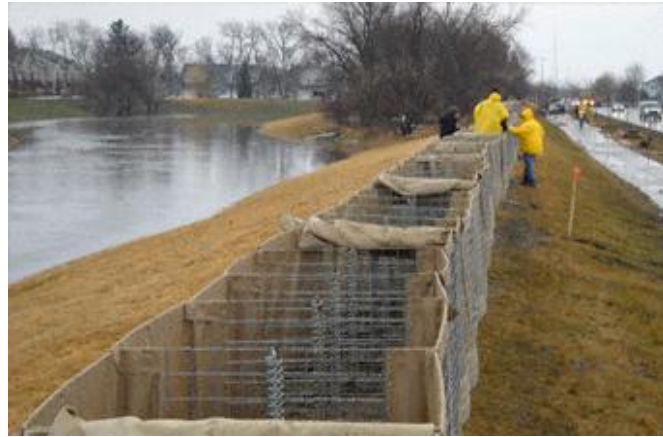
Figure 24. HESCO Floodline Concertainer Installation
