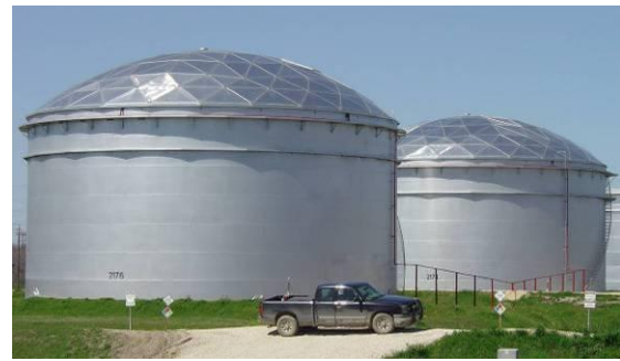
Figure 6. Wind Girders on Tanks
