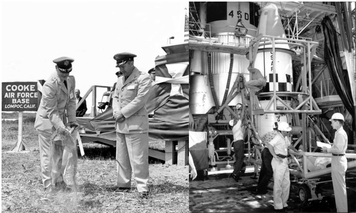
Left: Brigadier General Osmond Ritland, then vice commander of WDD, breaks ground at Cooke AFB on 8 May 1957 for the construction of space and missile facilities on the west coast. Cooke was soon renamed Vandenberg AFB. Right: Officers of AFBMD's 6555 th ATW discuss their final inspection of the Agena spacecraft (in cradle) for the launch of MIDAS 2 on Atlas 45D (in background) on 24 May 1960.
