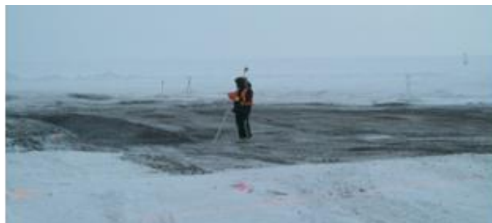
Surveys are done before work starts
