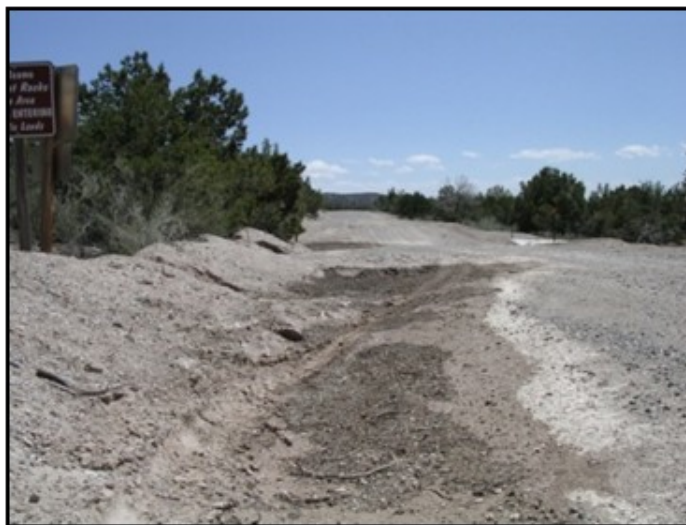
This road to the monument will be improved.
