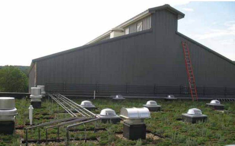
The roof (in the foreground) of the Armed Forces Reserve Center and Field Maintenance Shop in Mount Carmel, Tennessee is covered with vegetation to help cool the building and keep utility costs down.
