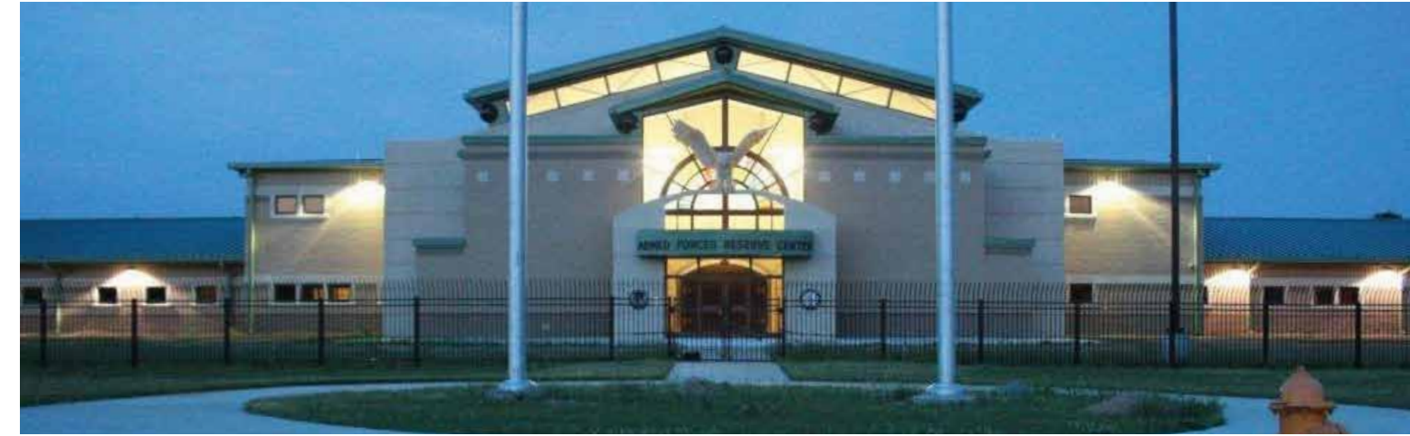
The new Armed Forces Reserve Center in Mt. Vernon, Illinois is heated with geothermal heat pumps.
