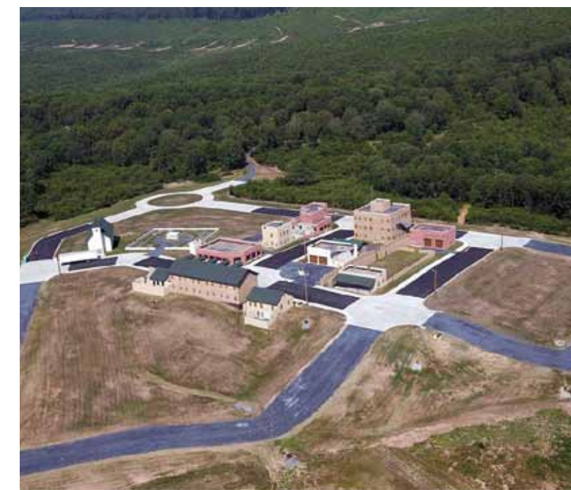
The 50-acre Combined Arms Collective Training Facility (CACTF) at Fort Indiantown Gap consists of 11 concrete buildings that simulate an Iraqi village—complete with a mosque, a police station, a gas station and a dormitory. Photo by Robert Smith.
