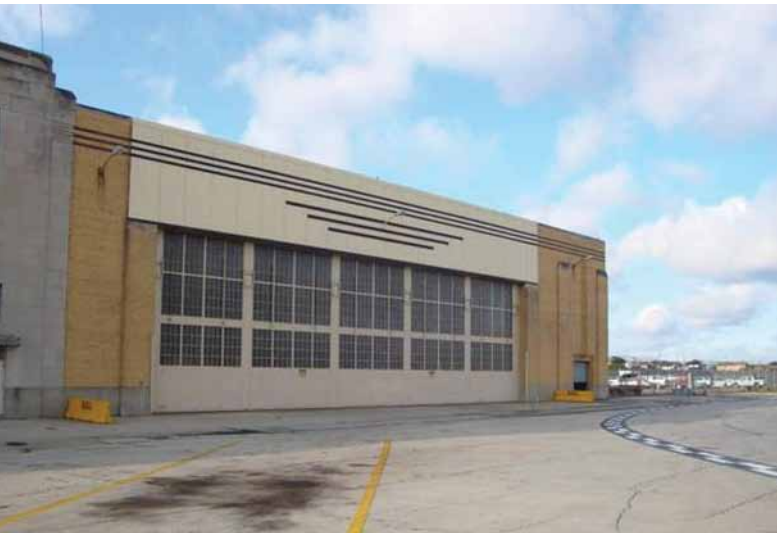
Due to runway extensions and the increased size of commercial airliners, the safety zone between the apron of the Army Aviation Support Facility (AASF) in Kankakee, Illinois and the adjacent Greater Kankakee Airport taxiway has become so short that the wings of commercial aircraft enter into the AASF apron air space while taxiing. This is considered to be a high safety risk for Soldiers and civilians. In addition, training capabilities are hindered due to the short apron air space. The existing 48,161-square foot AASF was built in 1940.
