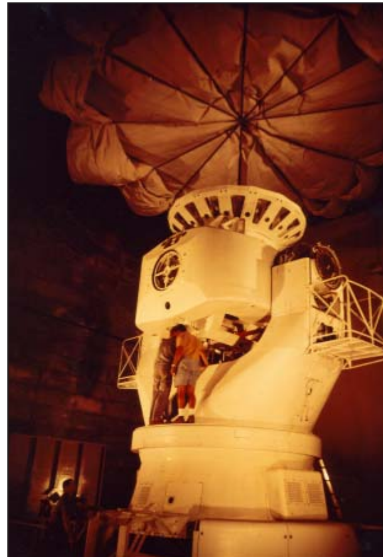
Installing the Radome on the Target Track Radar
