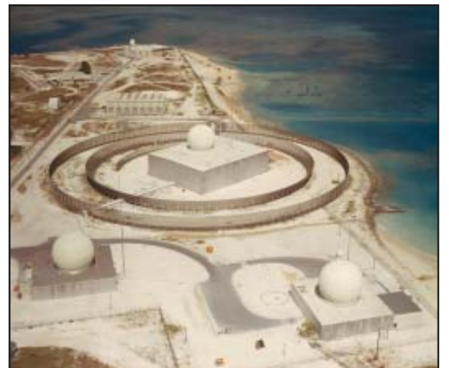
The Zeus Acquisition Radar and smaller Target Tract Radars on Kwajalein Island, Republic of the Marshall Islands
