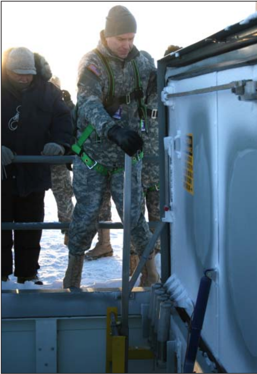
Braving the frigid temperatures of 40 below zero, Brig. Gen. James W. Nuttall, deputy director of the Army National Guard, descends into a Silo Interface Vault on the Missile Defense Complex on Fort Greely.
