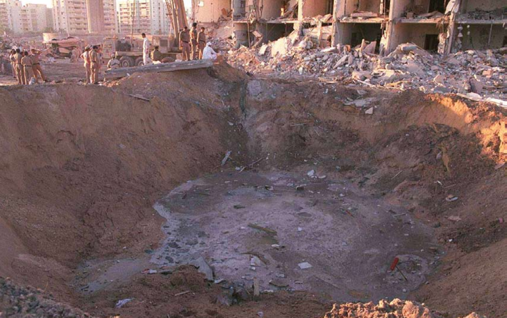
Ground Zero at Khobar Towers. (DOD image taken 6/26/96. Photographer unknown.)
