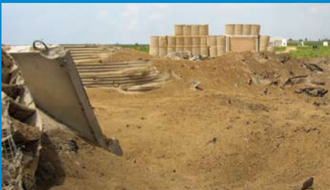
Fig. 5: The reaction structure used for testing pressure-sensitive laminate material survived two perimeter wall explosions.
