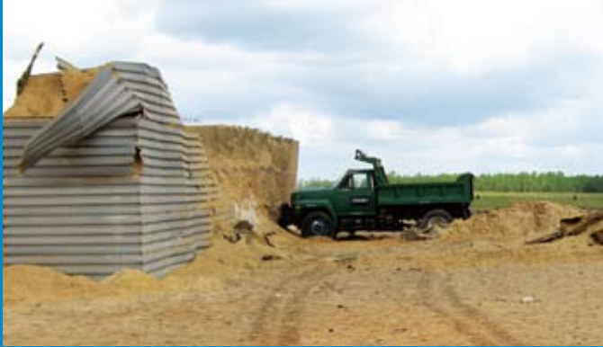
Fig. 3: Second vehicle test setup. The wire/fabric soil containers at left were most resistant to the effects of the first explosion. Note the damage to wall components.
