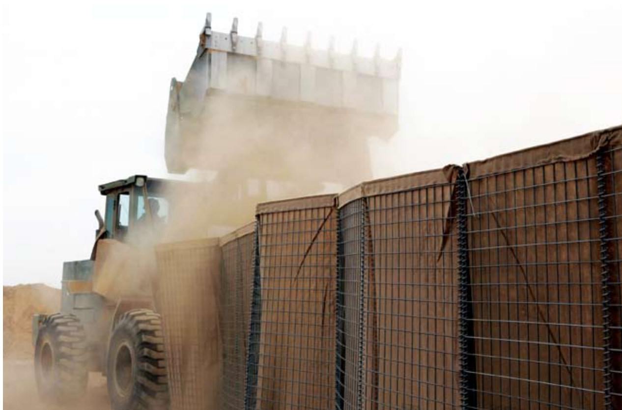
Fig.1 : Marines construct a combat outpost perimeter wall.
