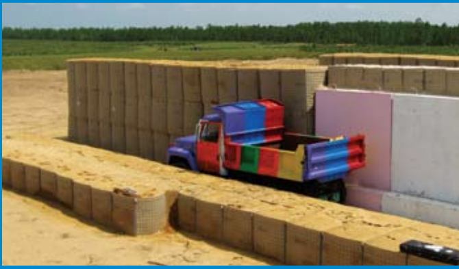
Fig. 2: Initial wall setup with first test vehicle. This setup allowed testing of a variety of wall configurations to determine the most effective design.
