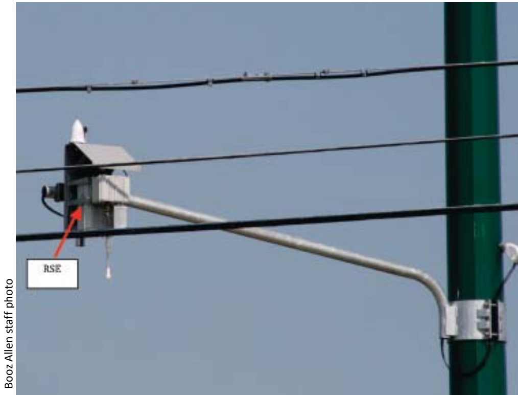
Figure 2-21: RSE Mounted to Pole in DTE
