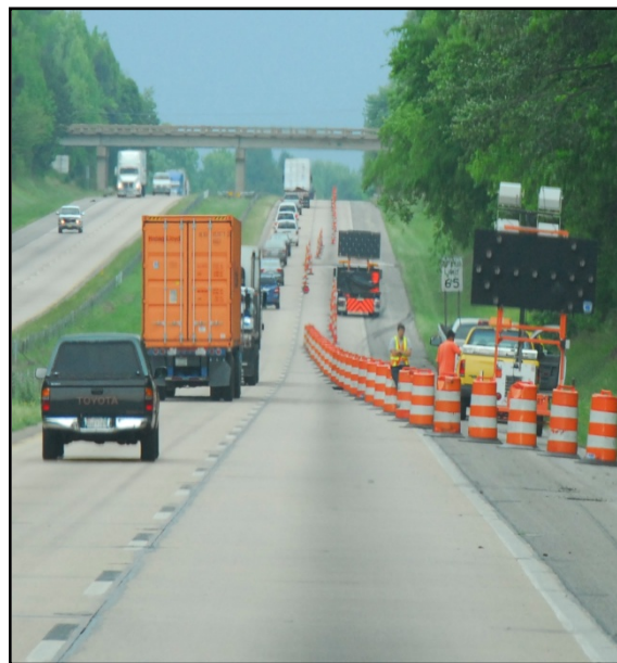
Figure 11. Work Zone in NC Where PTMDs Were Tested
