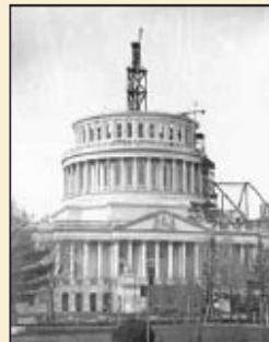
Construction of the new cast-iron dome was well under way in 1861 (left).
