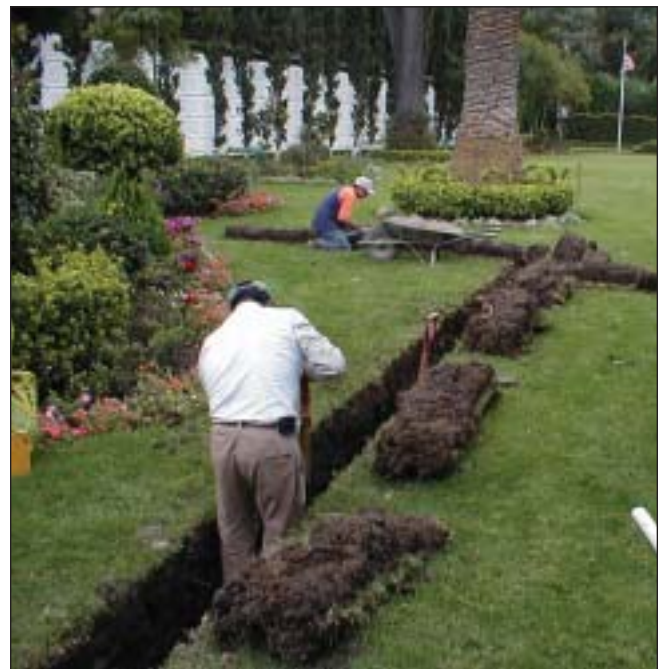
Workers install new sprinklers at Mexico City Cemetery
