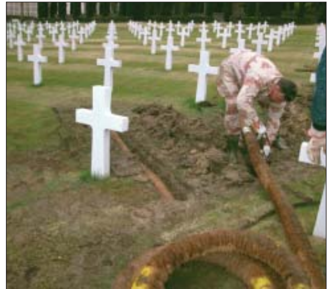
Drainage pipe is installed at Florence Cemetery
