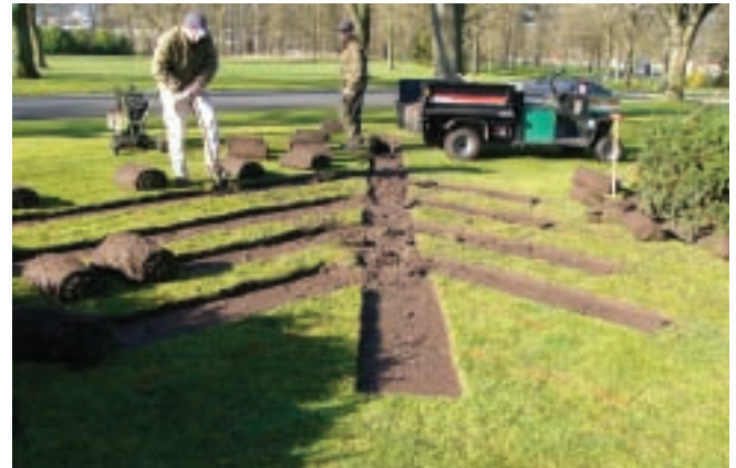
Working to improve soil drainage at Lorraine American Cemetery
