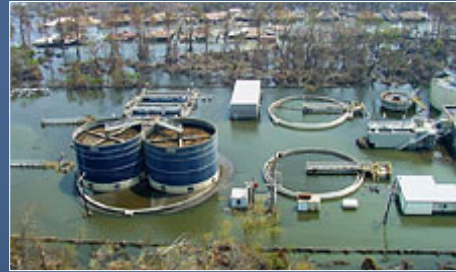
A wastewater treatment facility in St. Bernard Parish, Louisiana. Photo by Louisiana DEQ
