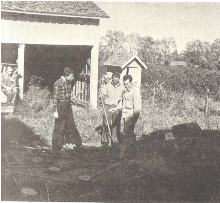
The Construction Situation
