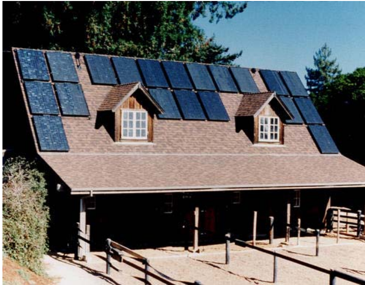
Figure 18. Solar-powered horse corral. Source: NREL PIX.
