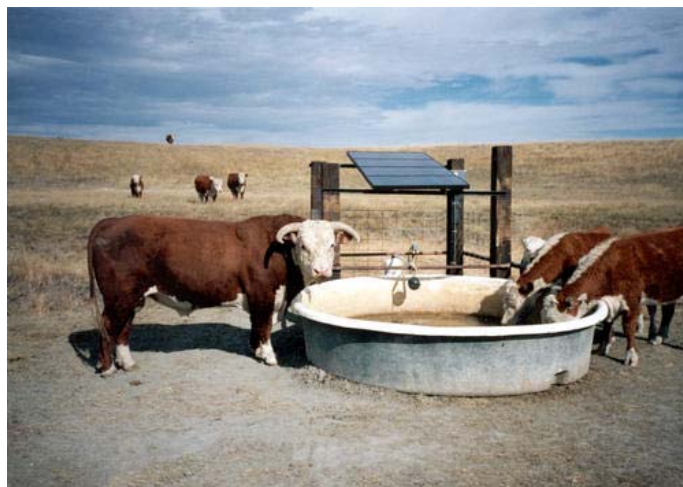
Figure 19. Solar-powered water pumping station. Source: NREL PIX.
