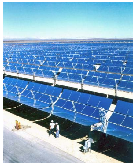
Figure 21. Parabolic trough solar power facility. Source: NREL PIX.
