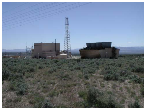
Figure 36. Single flash geothermal power plant. Source: NREL PIX.
