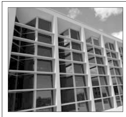
The Trombe wall at the NREL Visitors Center in Golden, Colorado, provides passive heating and daylighting to the exhibit hall.
