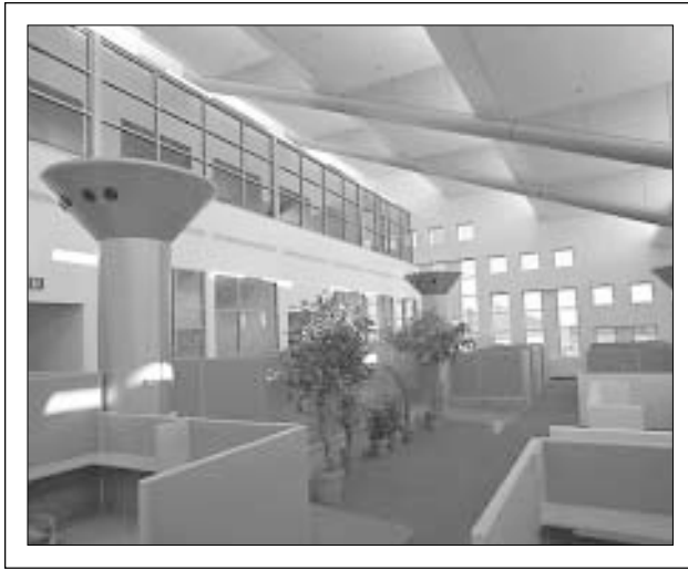
Each innovative “air tree” above provides ventilation for six offices at the National Renewable Energy Laboratory’s (NREL’s) Solar Energy Research Facility in Golden, Colorado. Air is cooled and humidified by direct evaporation, or “swamp cooling.”
