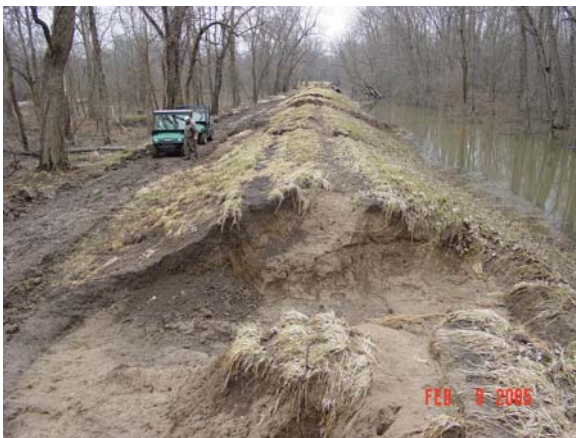
Figure 6.2 and 6.3, Levee breaches along the Wabash River
