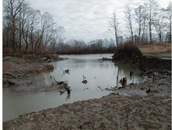
Figure 6.1, Levee breach in Lynden, WA
