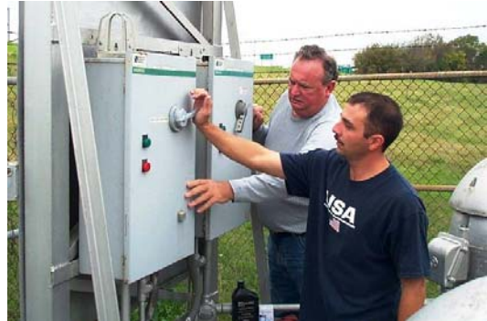
Figure 7.1. Inspection of pumping station controls. (OK)
