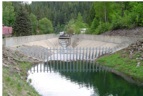
Figure 2.73 ACCEPTABLE intake structure upstream of the concrete channel. (ID)
