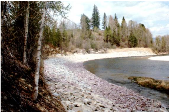
Figure 2.25 ACCEPTABLE riprap for erosion control. (MT)
