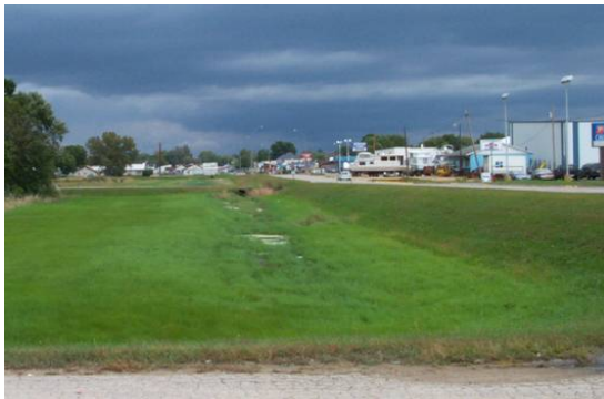
Figure 2.54 ACCEPTABLE interior drainage channel. (IA)
