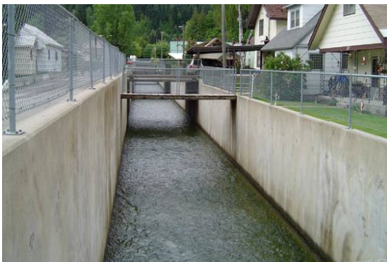
Figure 2.72 ACCEPTABLE concrete lined flood control channel. (ID)
