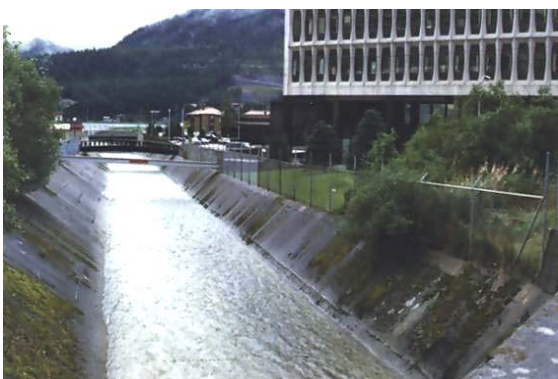
Figure 2.74 ACCEPTABLE concrete lined channel. (AK)
