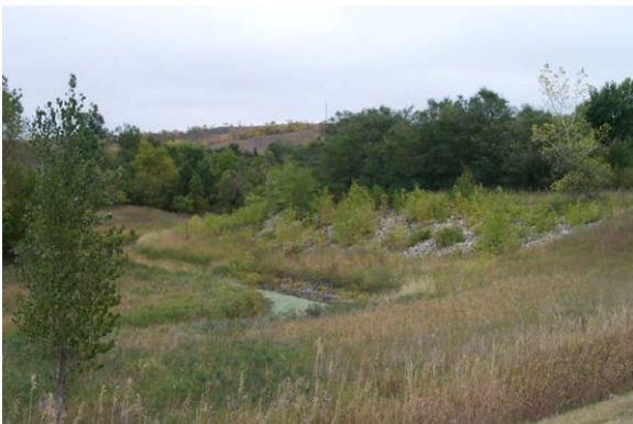
Figure 2.27 MINIMALLY ACCEPTABLE. Trees and saplings are becoming established within riprap-protected areas and along the lower portions of the river channel, and must be removed. (ND)
