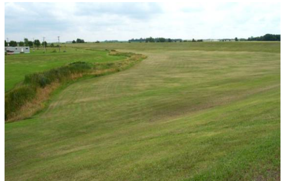
Figure 2.57 ACCEPTABLE interior ponding area and drainage ditch. (MN)
