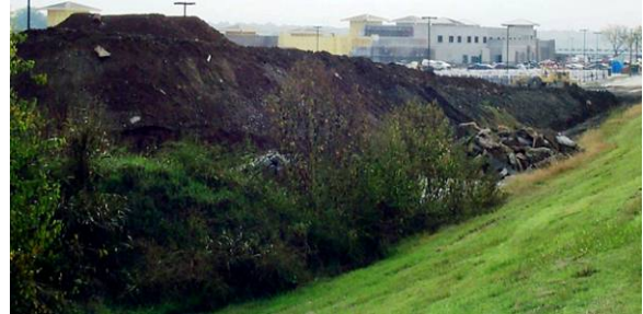
Figure 2.10 UNACCEPTABLE, unapproved encroachment. Material stockpiled against the levee. (OK)
