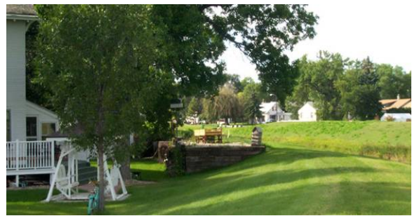
Figure 2.14 UNACCEPTABLE encroachment. Patio construction using railway timbers and fill without approval. (ND)
