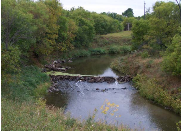
Figure 2.21 Beaver dam. Such dams can stop flow within the channel and cause erosion to the channel banks. Sponsors are encouraged to remove beaver dams ASAP. (ND)
