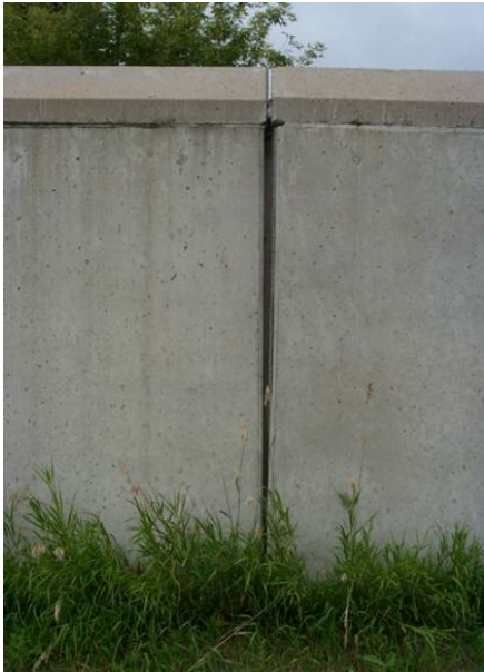
Figure 2.48 MINIMALLY ACCEPTABLE floodwall. Monolith joint separation caused by settlement, no landward or riverward tilting. The opening is about 3 inches wide at the top but the rubber joint sealer is still intact and undamaged. This joint has since been repaired by bolting another joint sealer on the both sides of the wall and filling the void with an expandable joint sealer. (ND)
