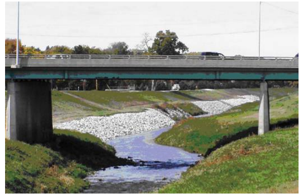
Figure 2.26 ACCEPTABLE riprap for erosion control. (NE)
