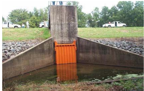
Figure 2.63 ACCEPTABLE culvert gate. (LA)
