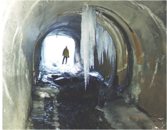
Figure 2.58 Concrete drainage tunnel. (AK)
