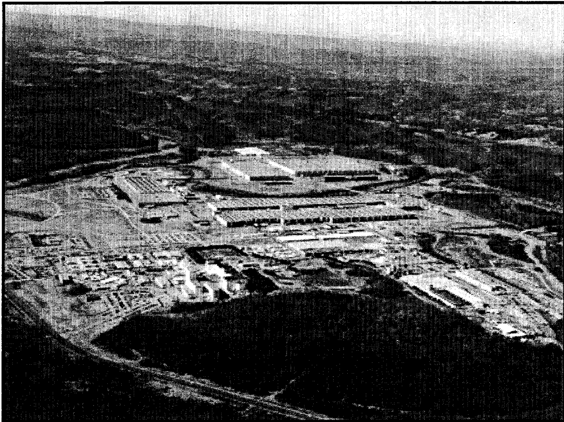
Figure 4.5 Aerial View of the Former K-25 Site Looking West
