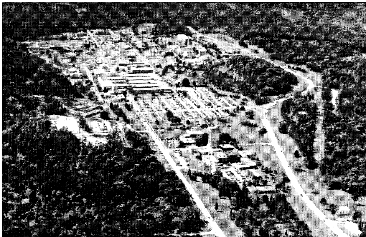
Figure 4.1 Aerial View of Bethel Valley Looking East
