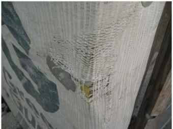
A transitional shelter constructed with thin plastic sheeting shows wear. (Photo by OIG, November 2010)
