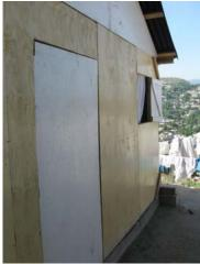
At left stands a transitional shelter built with plastic sheet walls, no solid doors, no windows, and no foundation. At right, an open window allows air to circulate in a transitional shelter built with plywood walls, doors, windows, and a concrete foundation. (Photos by OIG, November 2010)
